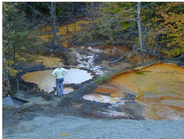
Figure 14.1.15-3: Iron Seeps Discharging at Base of TP-1, Elizabeth Mine
