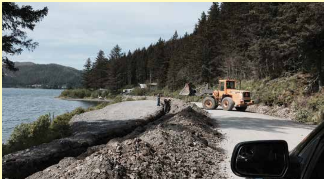
Workers dig to bury power lines in Cordova.
