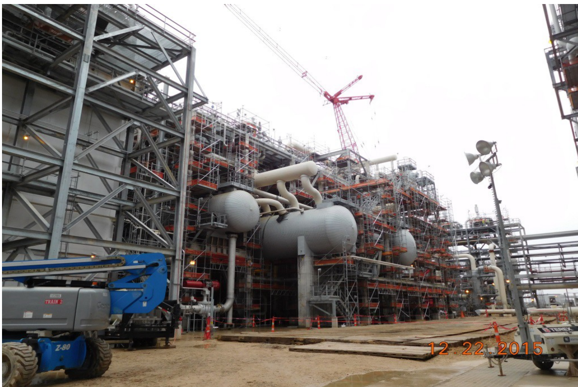
Train 2 – Pipe Installation in Propane Refrigeration Area
