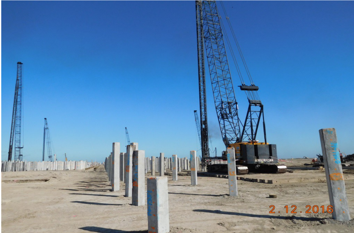
Train 5 Piling – Cryo Rack
