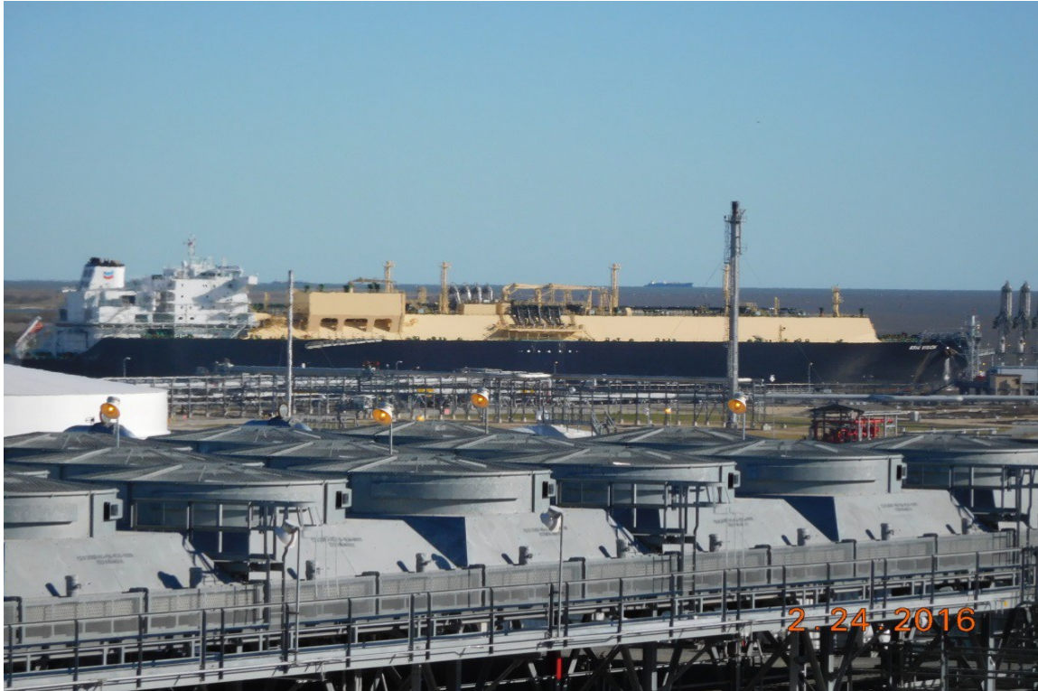
Train 1 – First LNG commissioning cargo being loaded into the LNG Carrier.
