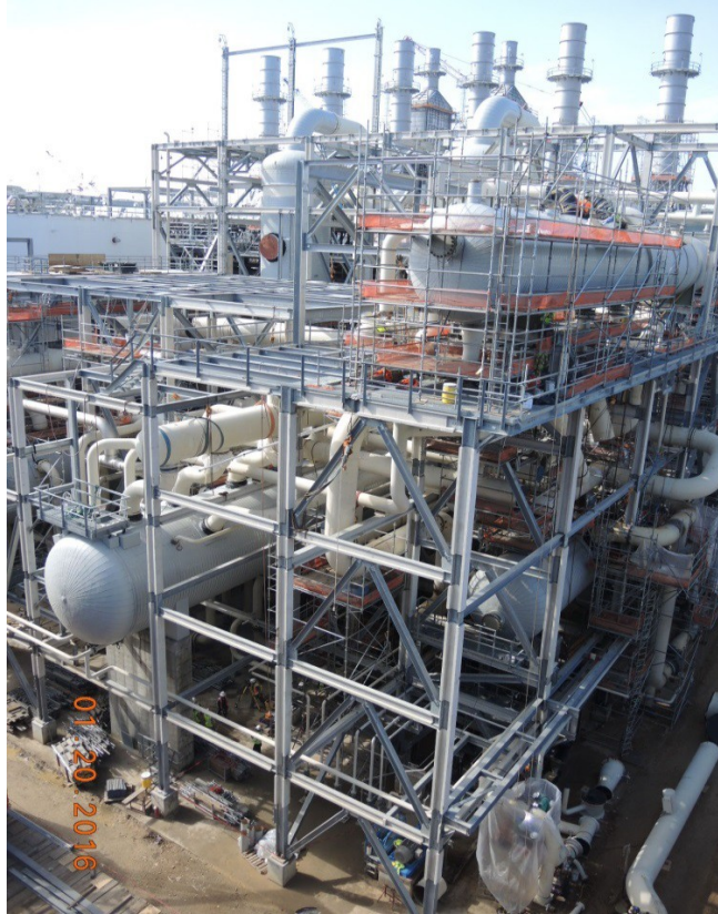
Train 3 – Erecting Steel in the Propane Refrigeration Area
