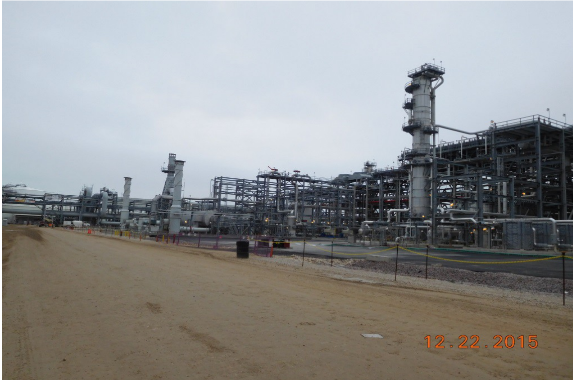
Train 1 – Looking down 1 st Ave; Purple Turnover Fences are Installed
