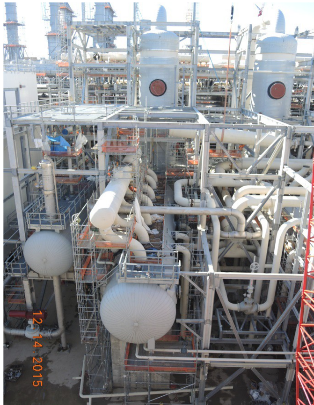
Train 3 – Installing Pipe in Propane Refrigeration Area
