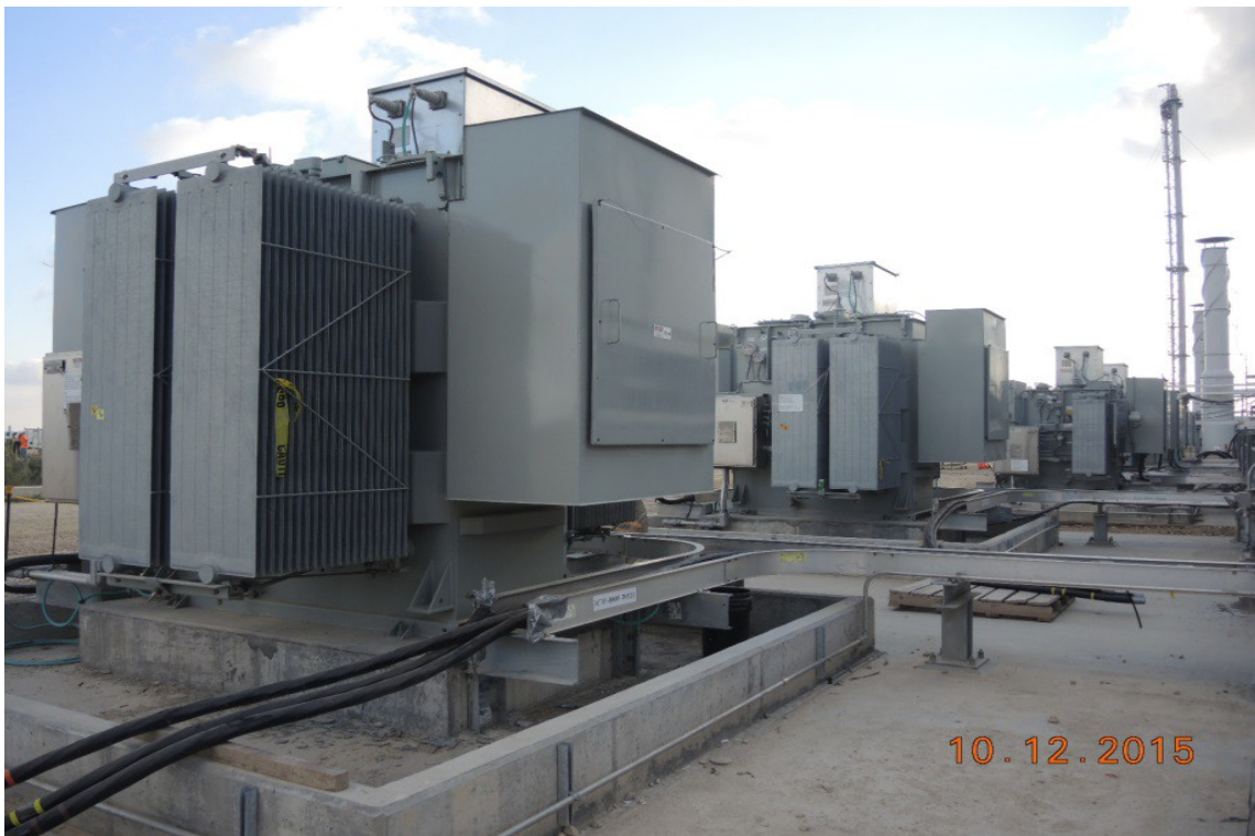
OSBL Pulling High Voltage Cable in the Utility Substation Area
