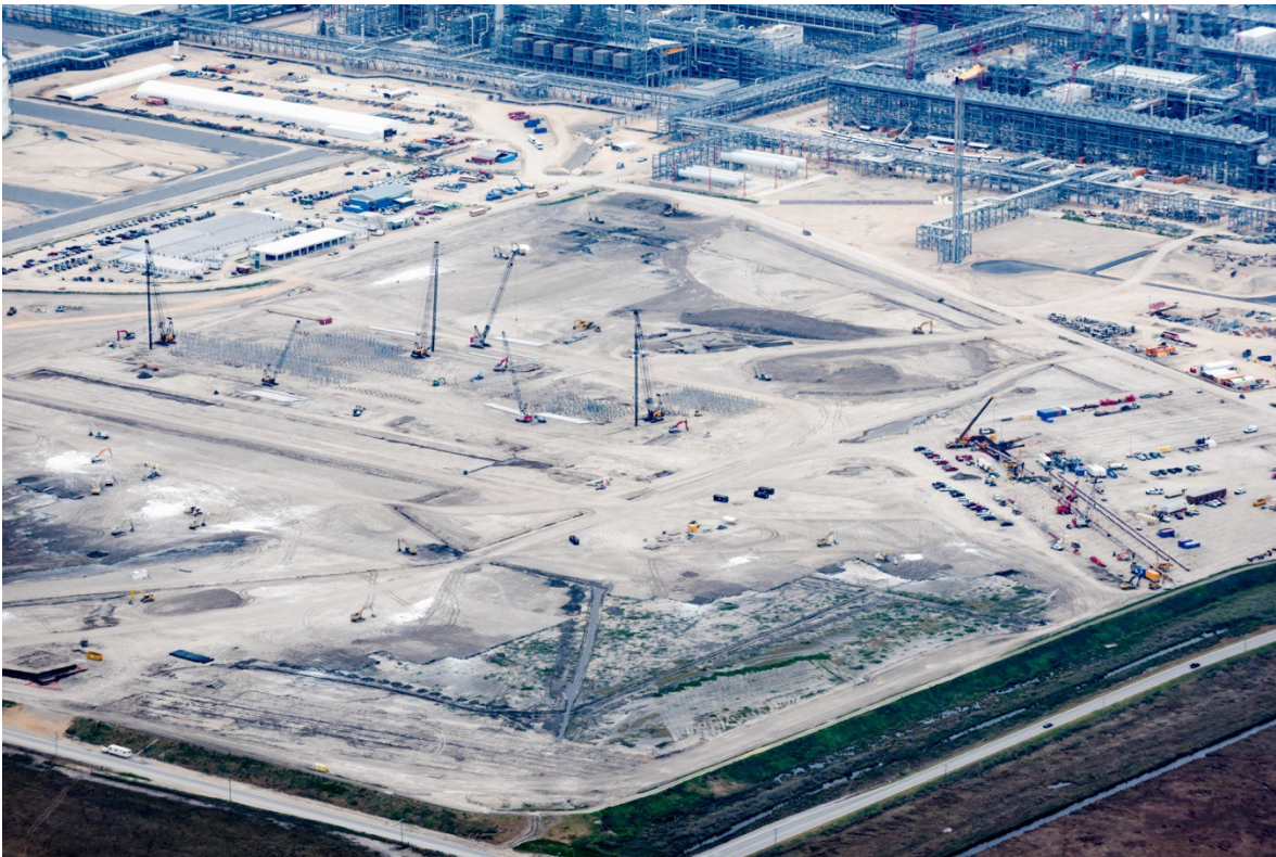
Stage 3 – Soils Improvement
