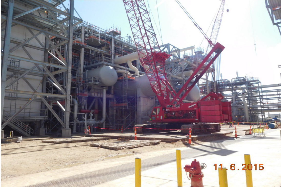
Train 2 – Installing Pipe in Propane Refrigeration
