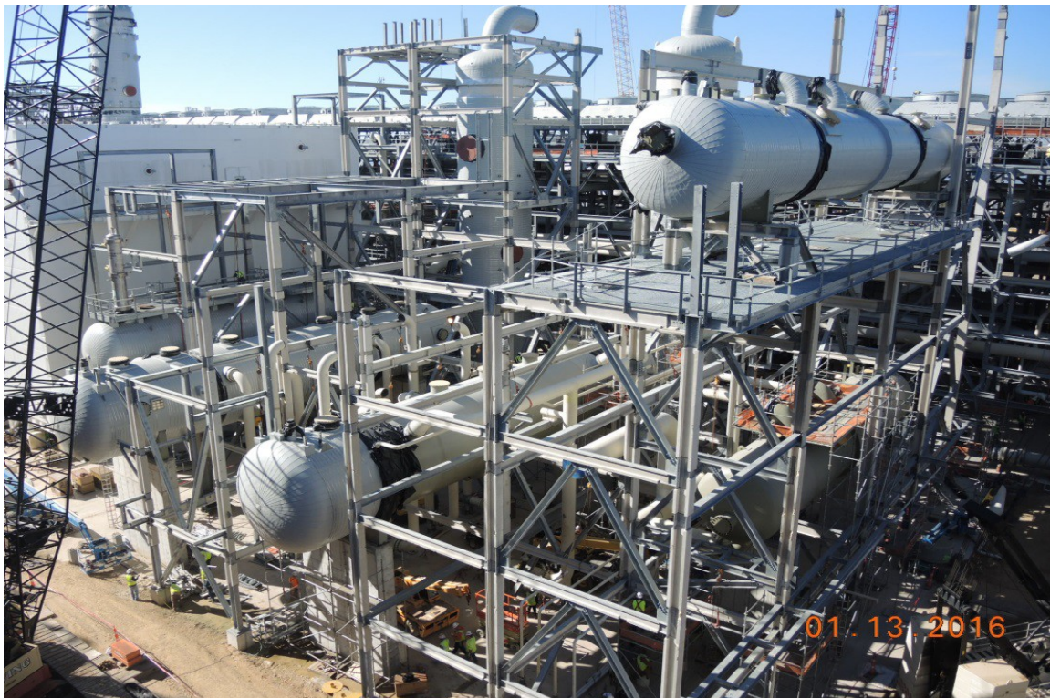
Train 4 – Erecting Steel in the Propane Refrigeration Area
