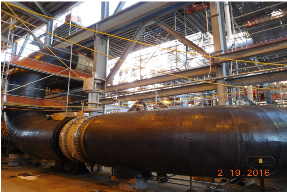
Train 2 – Insulating Large Bore Pipe on the Compressor Deck
