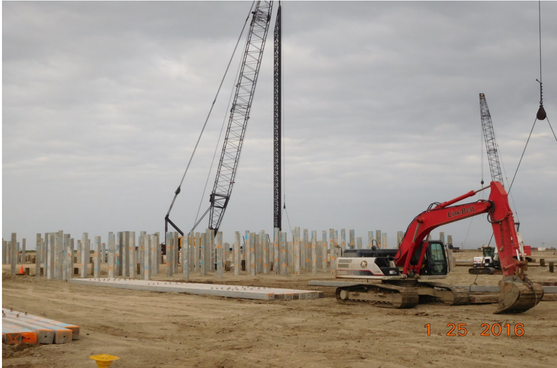
Stage 3 – Piling Progress
