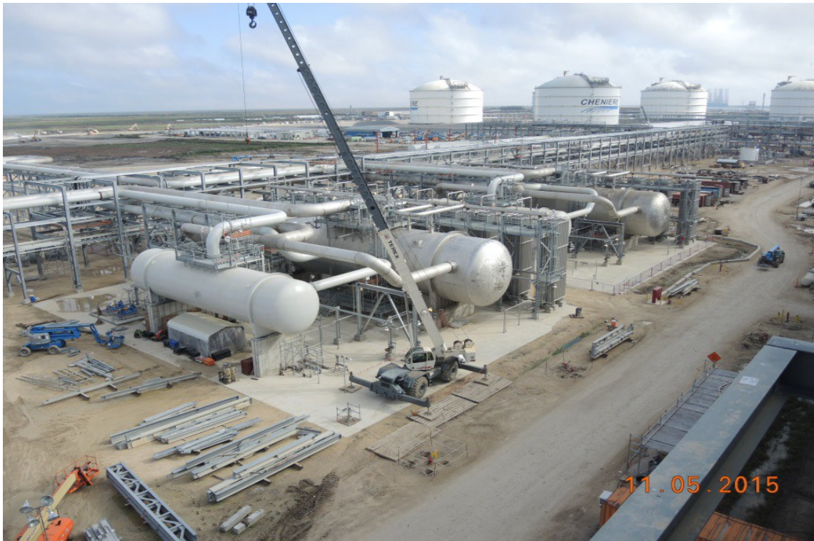
OSBL – Flare Knockout Drum
