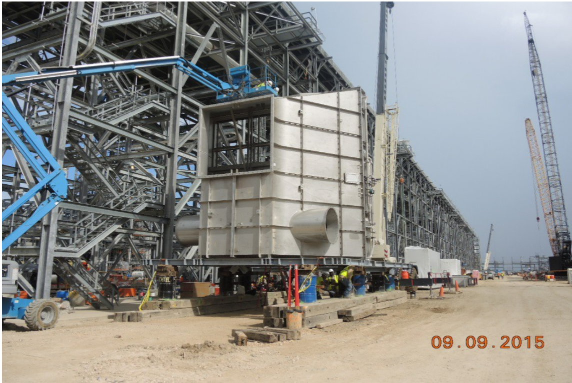
Train 3 – Compressor Area (Assembling Filter House)
