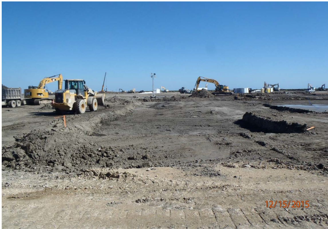
Stage 3 – Soil Stabilization Rough Grading in Train 5 area.
