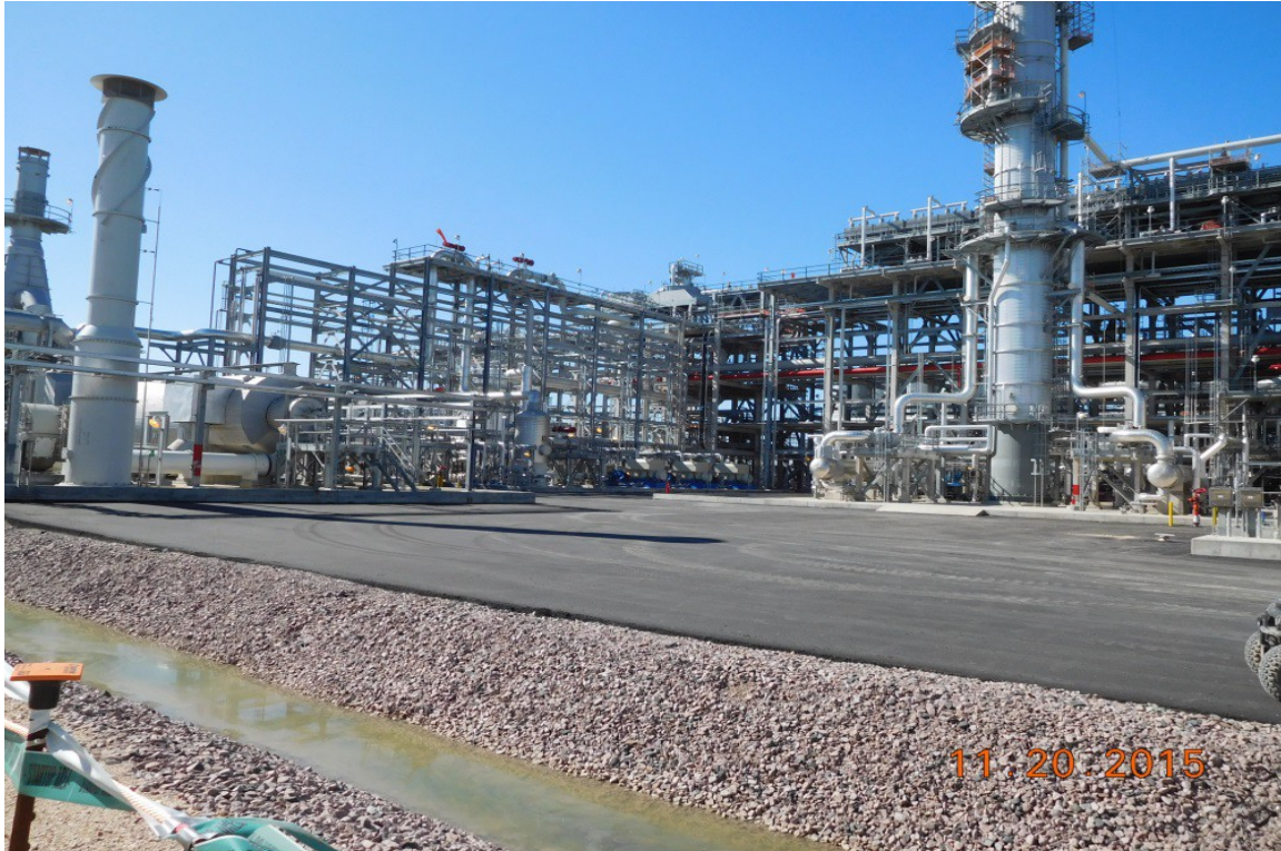
Train 1 – Asphalt Paving in Amine Regen and Acid Gas Removal Area
