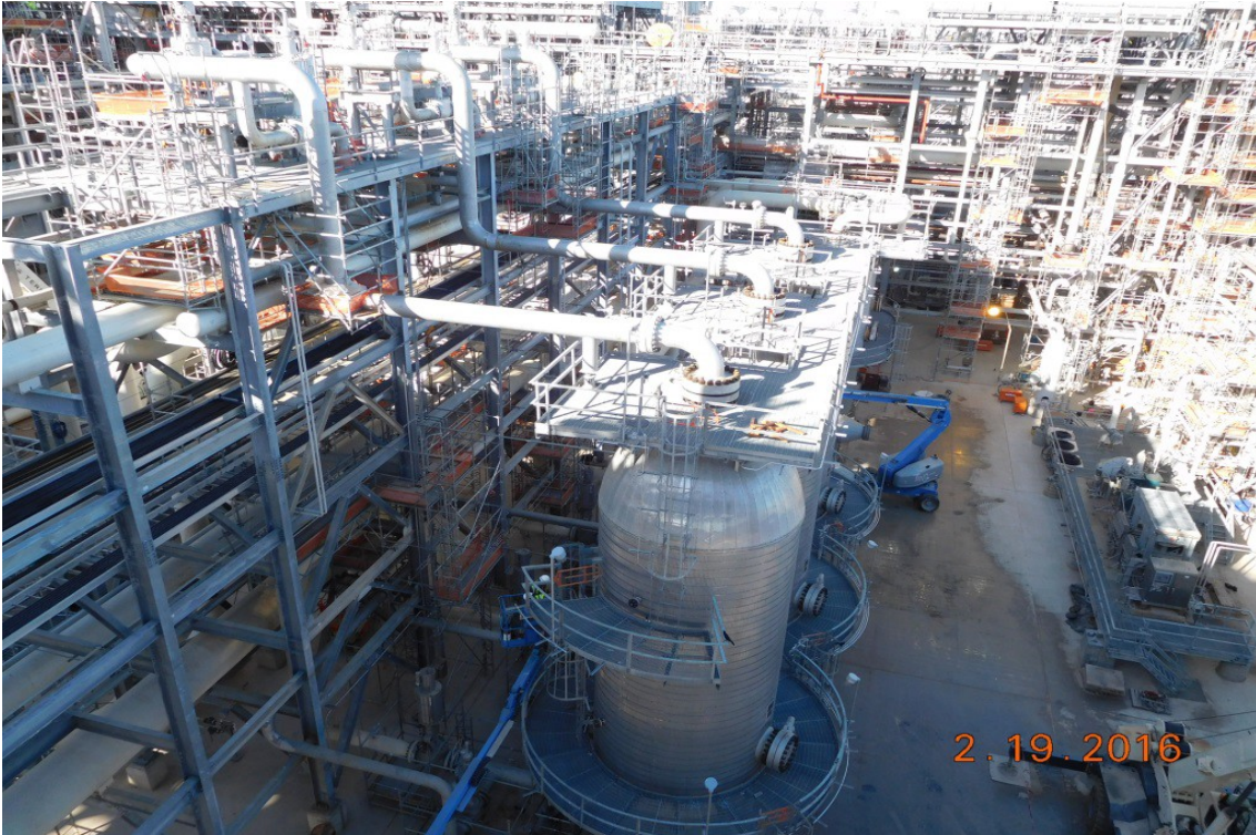
Train 3 – Molecular Sieve Dehydrators
