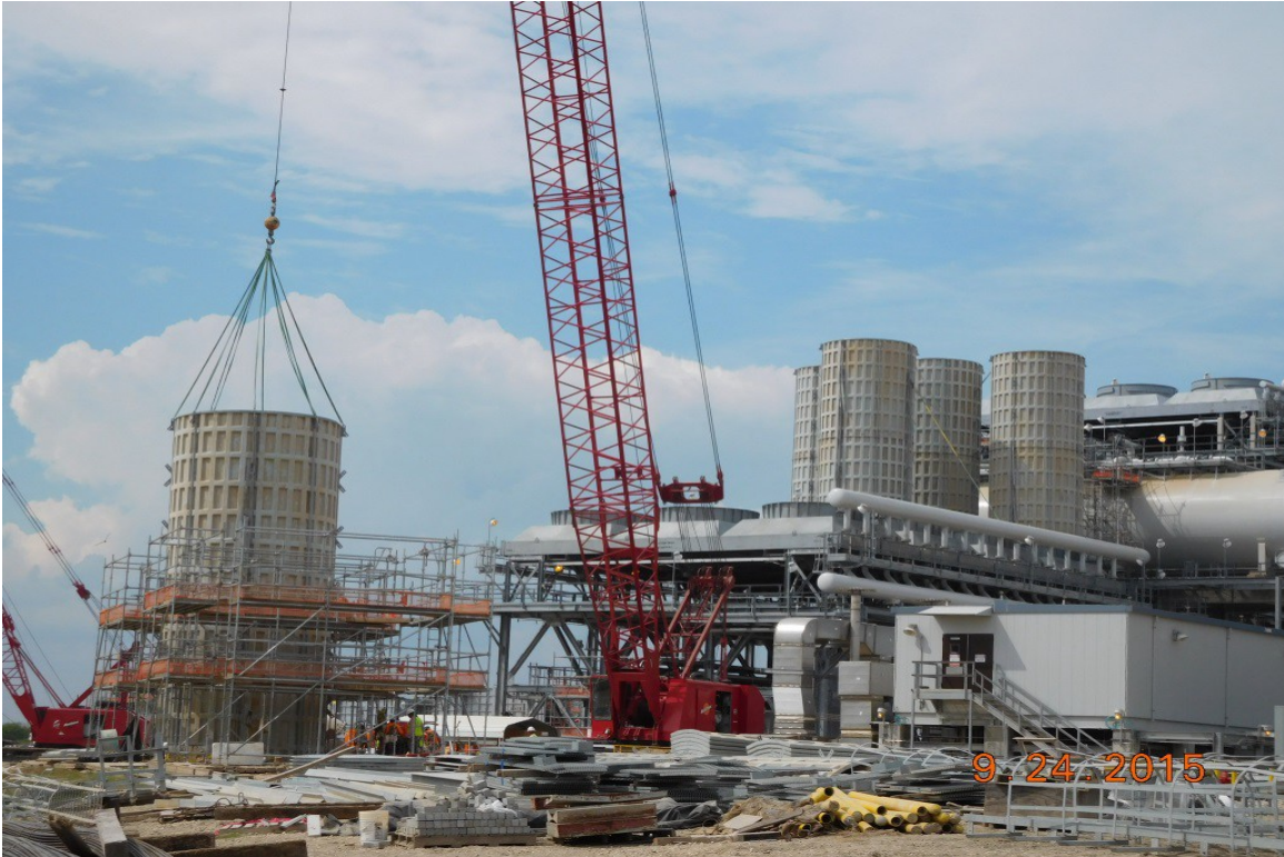
Train 2 – Setting Stacks in the Propane Refrigeration Area
