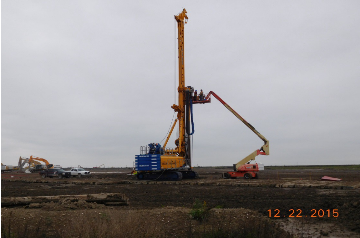
Stage 3 – Preparing Equipment for Piling
