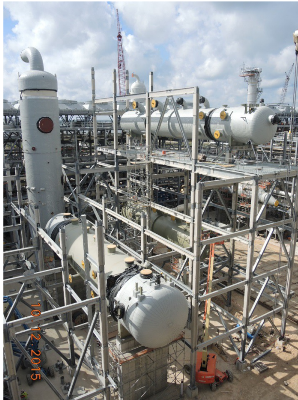
Train 4 – Erecting Structural Steel in Propane Refrigeration Area
