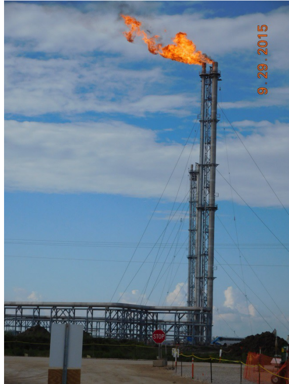
Train 1 – OSBL Lighting of Flare
