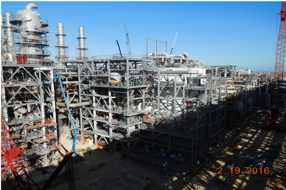
Train 3 – Ethylene Cold Box Structure Progress
