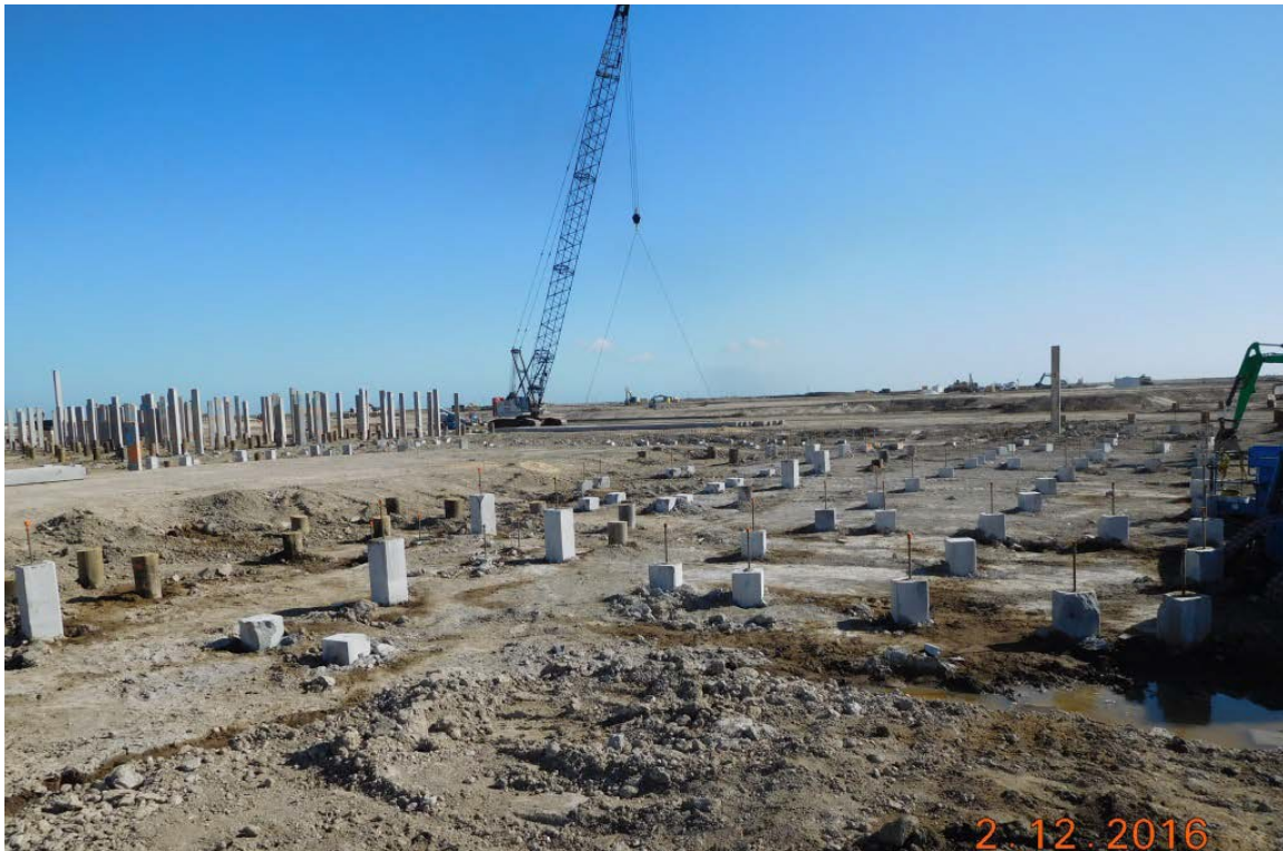
Train 5 Piling – Pile Cutting and Tension Connector Installation in Amine Area
