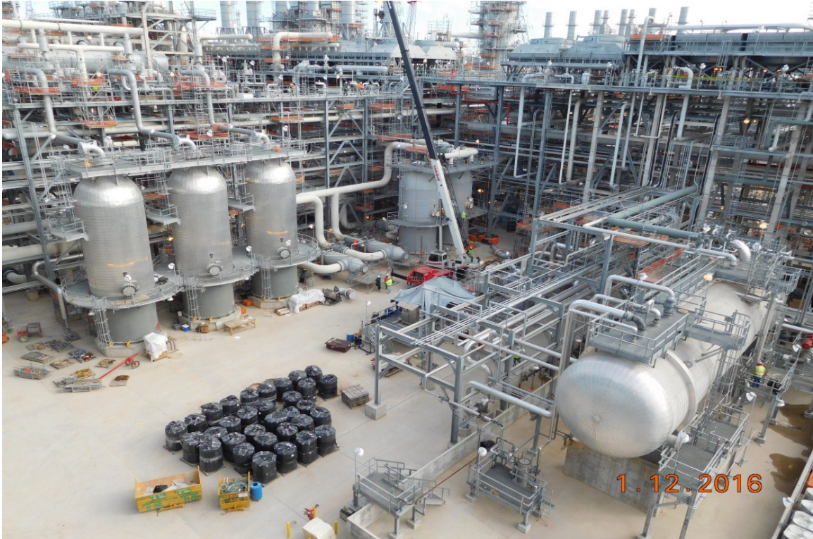
Train 2 – Prepare to Load Internals in Mercury Removal Beds
