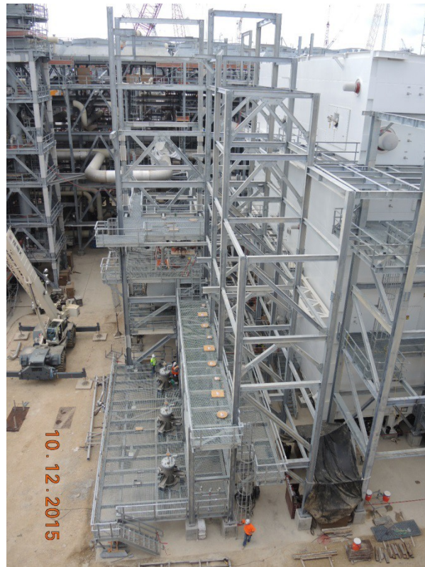
Train 3 – Erecting Structural Steel in the Ethylene Cold Box Area
