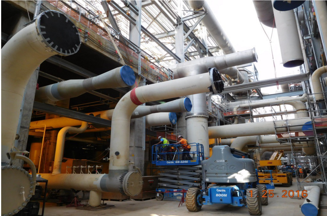
Train 3 – Installation of Refrigeration Piping in the Alleyway
