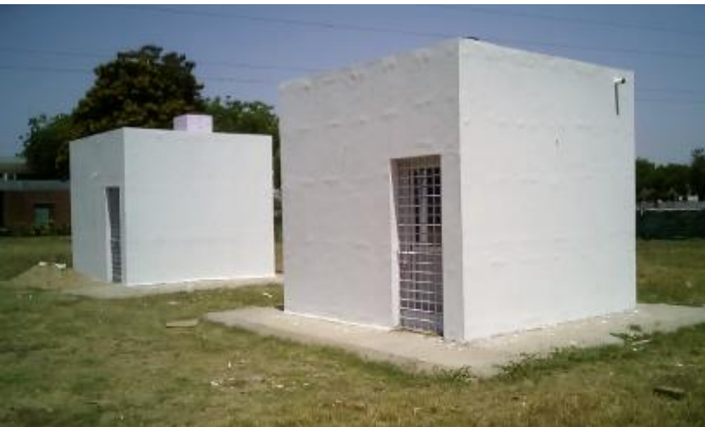
Measurement of performance of ceiling tiles made of new phase change materials in test bed, in naturally ventilated and forced ventilation modes.
