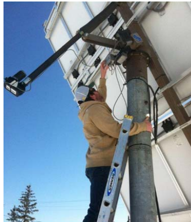
Photo by Brian Hirsch, NREL 20893
