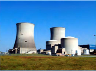
Watts Bar Nuclear Plant
