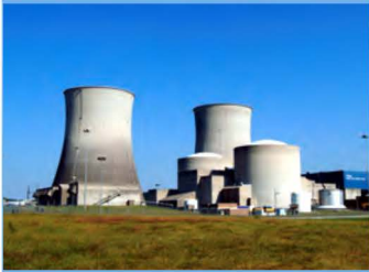
Watts Bar Nuclear Plant
