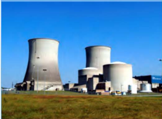
Watts Bar Nuclear Plant
