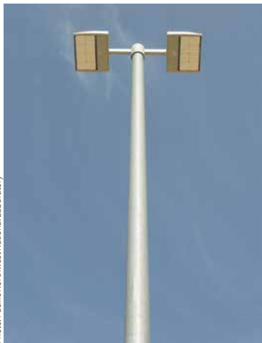
Quartz metal halide fixtures (top) were replaced by LED luminaires (two per pole) on the U.S.-Mexico border.
