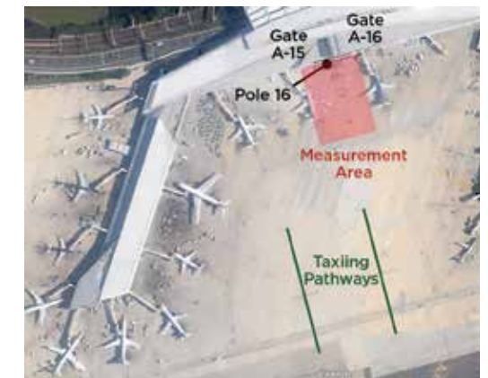
An aerial view of Terminal A, where the trial LED installation took place in the apron area immediately in front of Pole 16.
