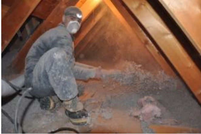
Blowing in cellulose in the village store
