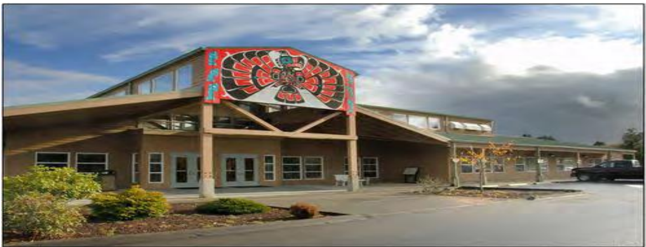
Figure 6: QIN Administrative Complex to be heated by Biomass for Heat Facility
