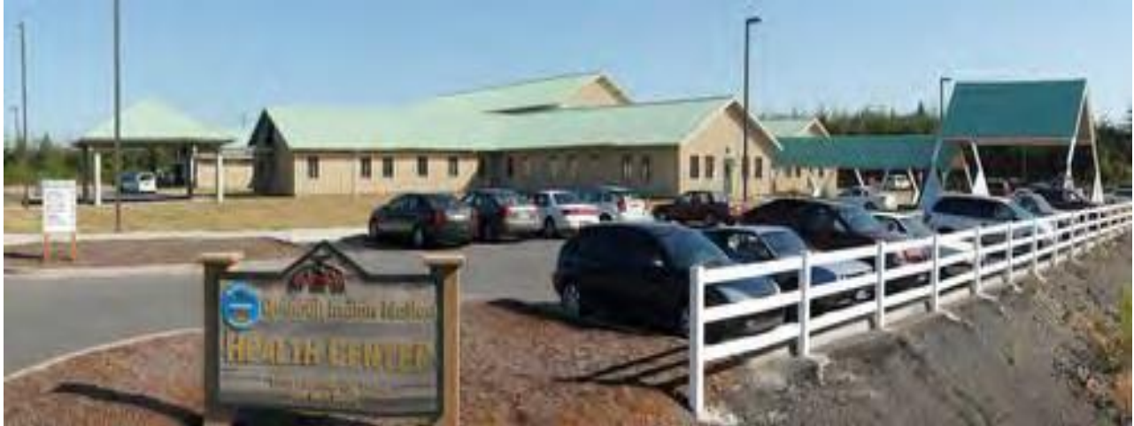
Figure 7: QIN Roger Saux Health Clinic to be heated by Biomass for Heat Facility
