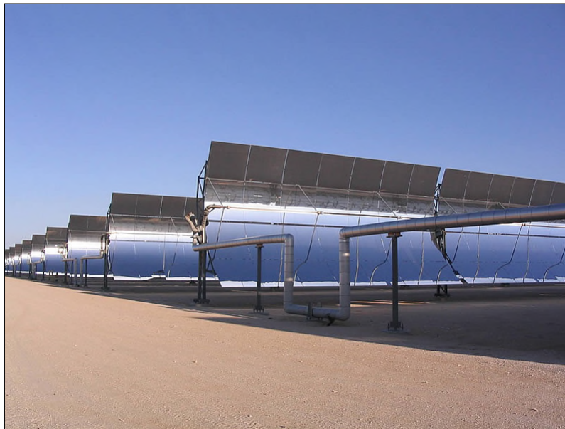
Figure 2-19. Concentrating Solar Thermal Power: 80-MW Solar Energy Generating Station (SEGS-IX) in Kramer Junction/Harper Lake, California
