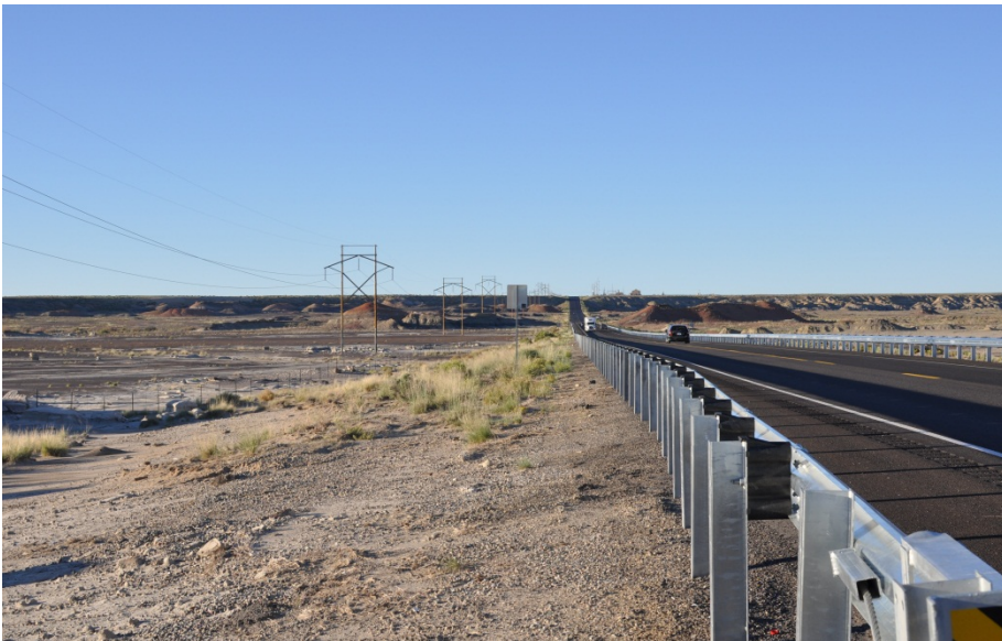
Photograph 38. View of transmission line from area below the Bisti Natural Gas Compressor Station along Highway 371 (not pictured but to the east), looking north. Bisti Substation is shown in the distant background.
