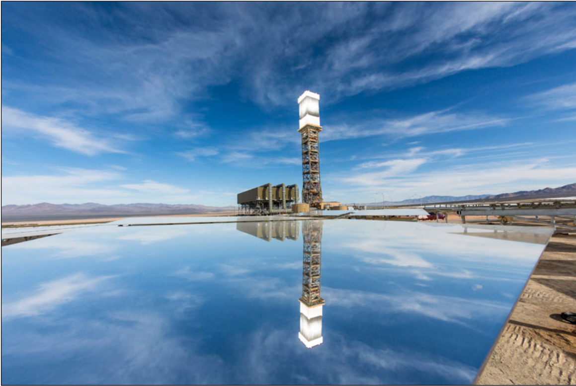
Figure 2-20. Concentrating Solar Thermal Power: The Just Commissioned (Feb 2014) Solar-Thermal Power Towers at Ivanpah, California, 392-MW Total Capacity
