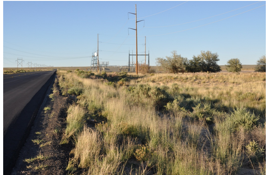
Photograph 44. View of potential Site 1A and Bisti Substation from area between the Substation and the Natural Gas Compressor Station along Highway 371, looking north.
