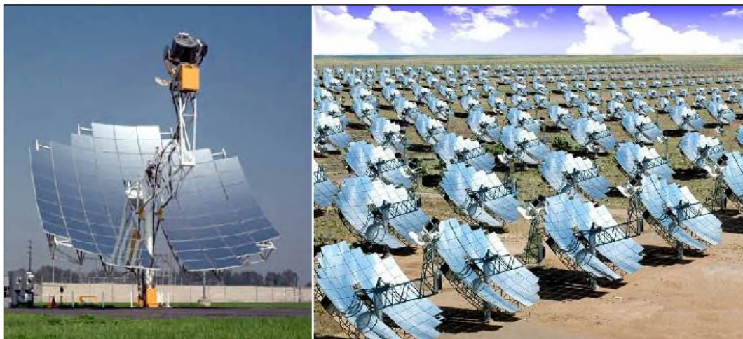
Figure 2-21. Concentrating Solar Thermal Power in Mojave, California: 10m-diameter 2-axis Tracking Dish with Stirling Engine at Focal Point
