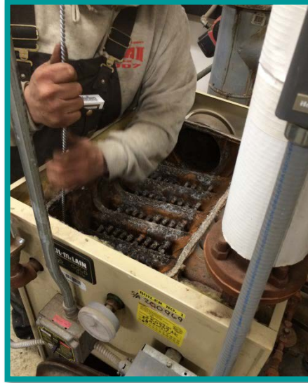
BEFORE: Brushing & cleaning soot from boiler
