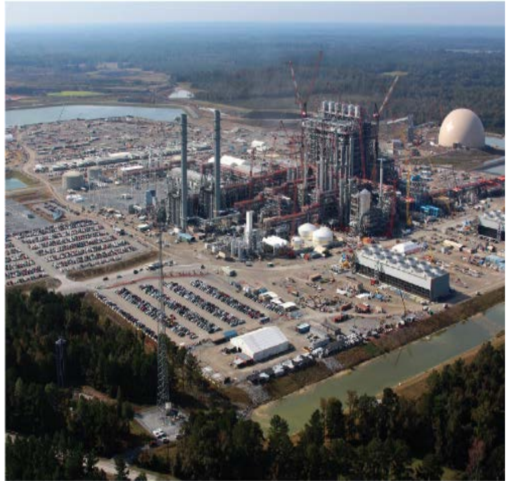
Southern Company Kemper Project, IGCC + CC + EOR Credit: Mississippi Power
