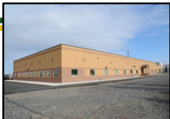
2009 Technical Support Building
