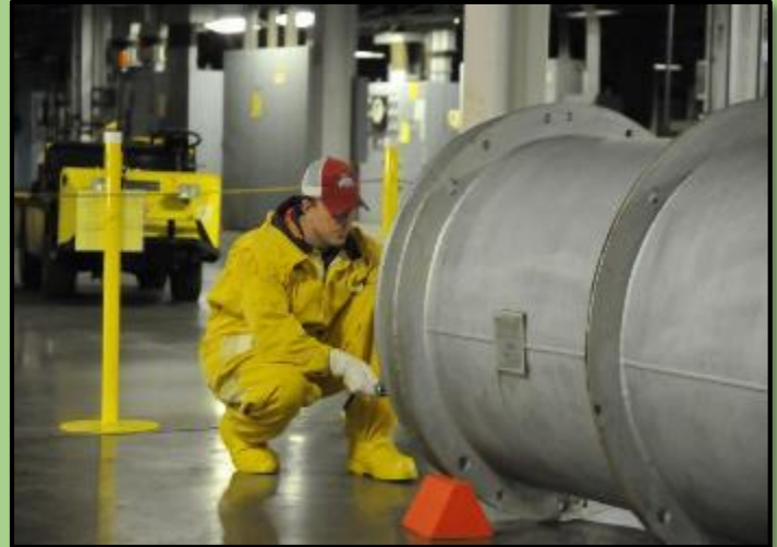
Cut-and-cap activities underway.
