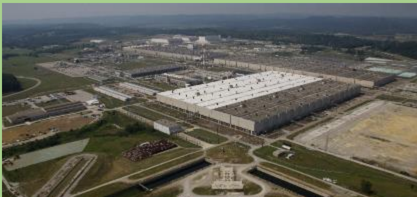
One of three former enrichment process buildings at Portsmouth.
