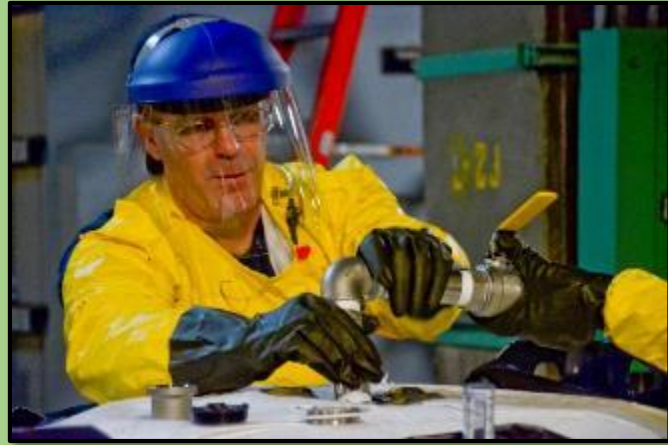
Worker removing PCB oil.
