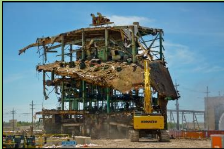
Demolition in progress at the C-410 UF6 Feed Plant.
