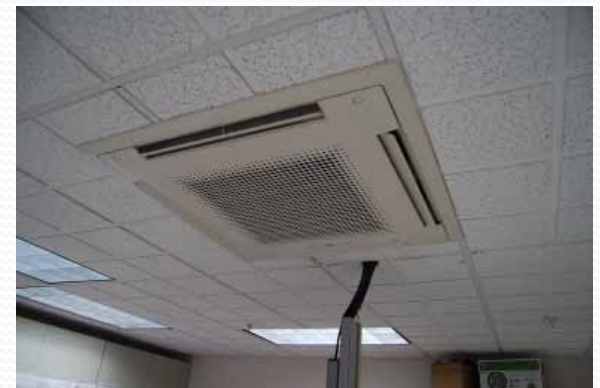
Ceiling Mounted Exhaust
