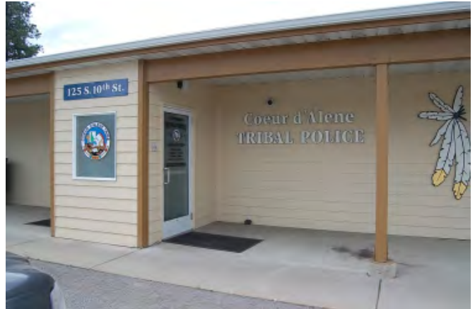
Figure 45. Tribal Police Headquarters entry.
