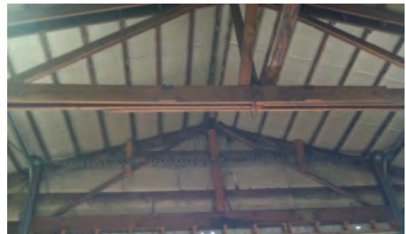
Figure 94. Integrated fiberglass insulation vinyl vapor barrier observed in ceiling and walls.
