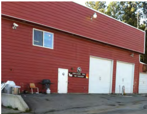
Figure 30. Fire Warehouse front entrance
