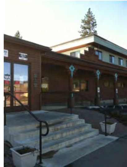
Figure 48. Old Benewah Medical Center front entrance with hydronic ice melt system embedded in sidewalk and steps
