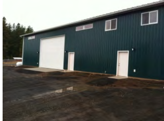
Figure 34. "New" Roads Maintenance Shop
