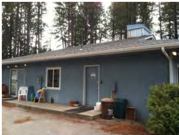
Figure 50. Youth Shelter entry.
