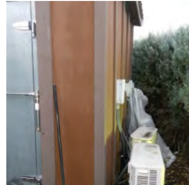
Figure 62. Kitchen air conditioning condenser units detailing potential impacts due to location
