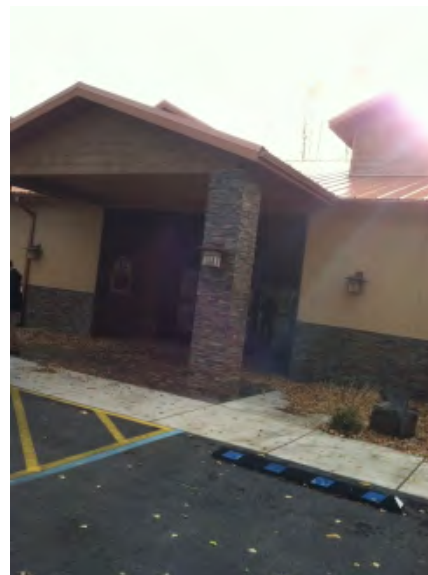
Figure 27. DeSmet Longhouse entry way
