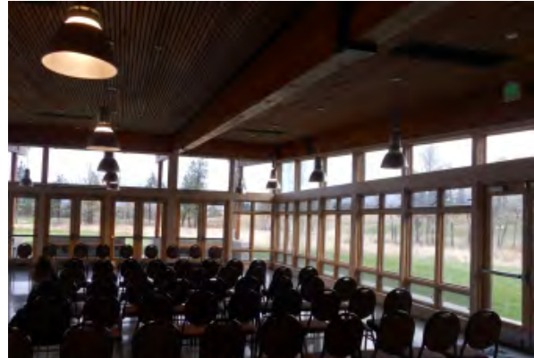
Figure 67. Pavillion interior showing suspended lighting and operable transom windows
