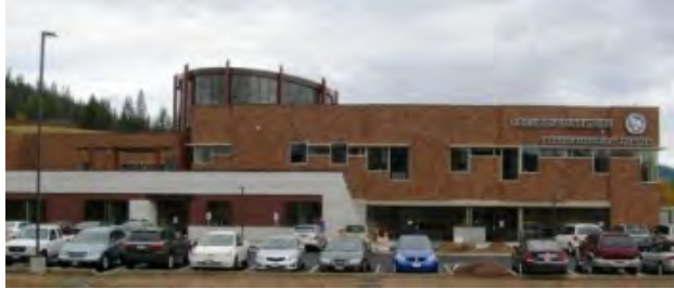
Figure 107. New Benewah Medical Center north facade.
