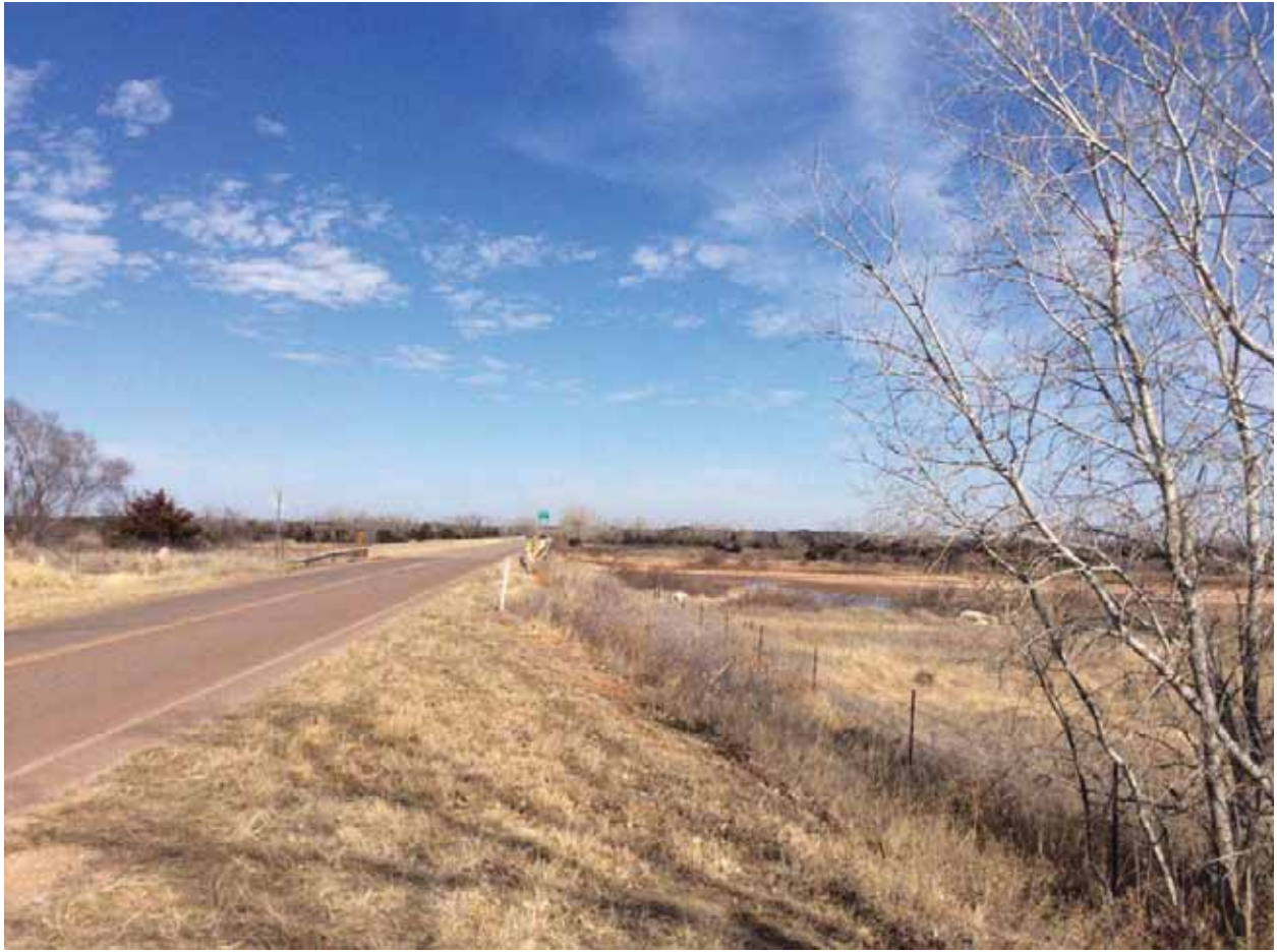
View northeast from the highway, crossing the Cimarron River. The area is rural with very little development near the river.
