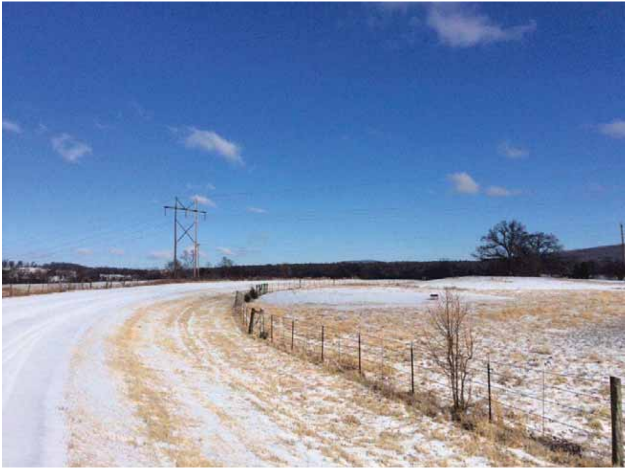
View northwest from Highway 352 and the historic Trail of Tears. There are single-family residences in the area and open fields in the FG.
