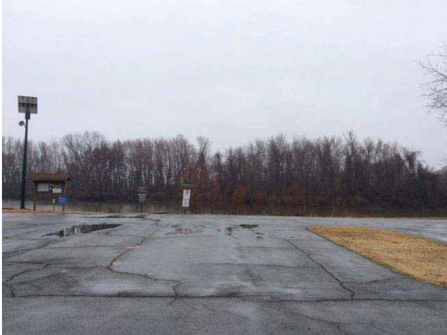
Views northeast (top) and north (bottom) from park and boat launch area. Views include wide section of stream, scattered trees and shrubs, parking lot, signs, vertical light poles, and dense line of trees along far stream bank. Large group picnic shelter and various smaller picnic areas are nearby.
