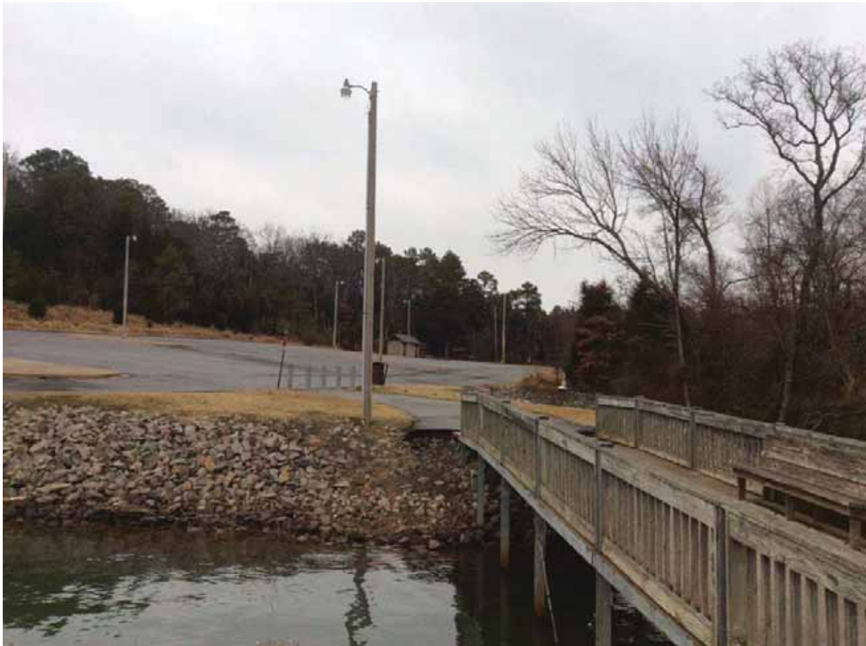
View north from boat launch area and fishing pier at lake on Lee Creek. Viewpoint includes wood light poles, parking lot, small restroom, and dense forest with mixed evergreen and deciduous trees. Because of the rising terrain to the north, an existing wood pole power line structure is barely visible.
