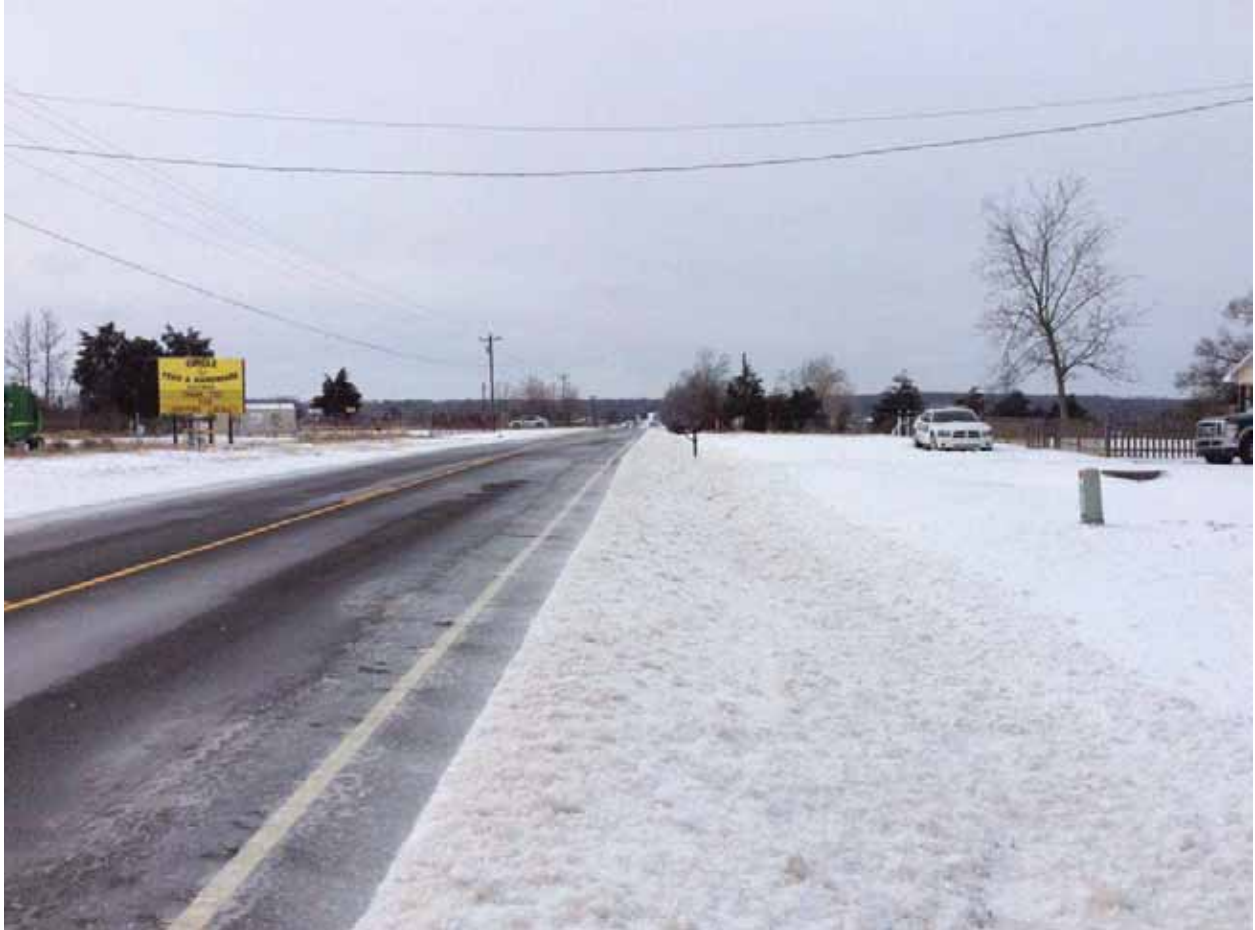
View south from the Highway 25 scenic highway. There are scattered rural residences and commercial buildings nearby and scattered to dense vegetation on both sides of the road.
