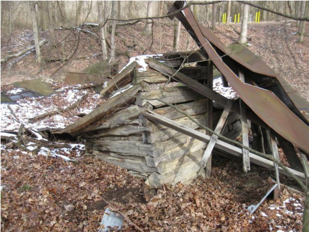
Figure 10. Photograph of the cabin (33Pk345) facing southeast.
