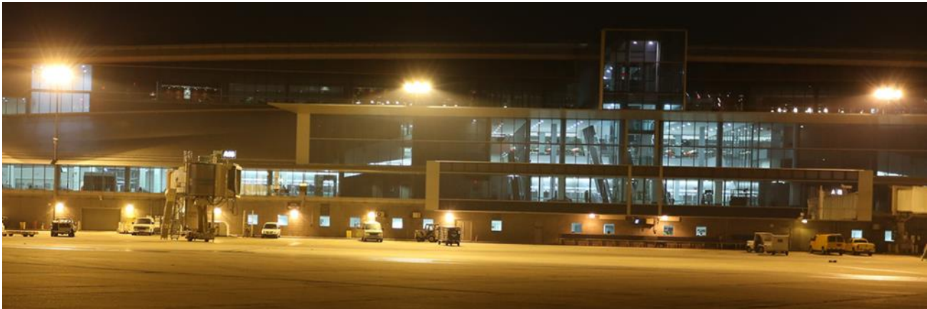
Figure 2. Photograph of the HPS system in the trial installation area. Pole 16 is at the center of the photo, with pole 15 to the left (west) and pole 17 to the right (east). The passenger boarding bridge serving gate A15 can be seen between poles 15 and 16.
