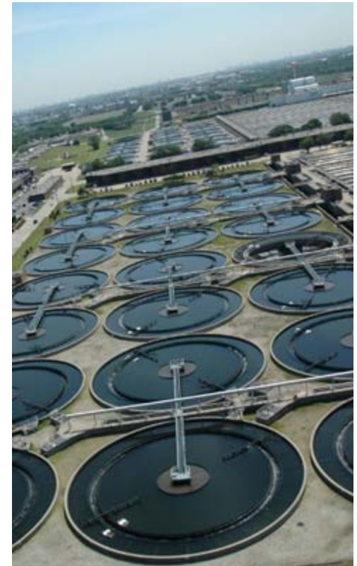
Stickney Water Reclamation Plant, Chicago
