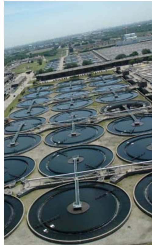
Stickney Water Reclamation Plant, Chicago
