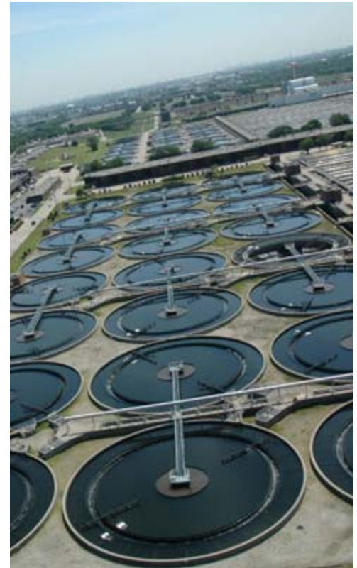
Stickney Water Reclamation Plant, Chicago
