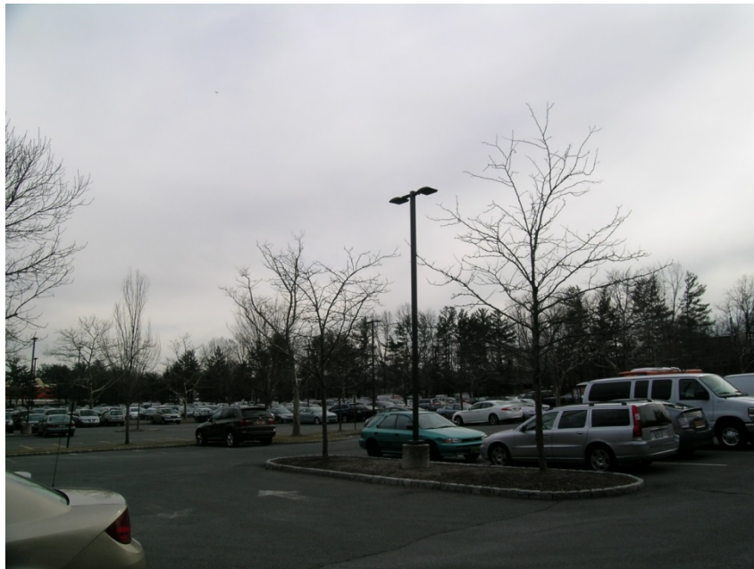
Figure 8: 15' poles with 100 W HPS lamps and 20' poles with 150 W HPS lamps.
