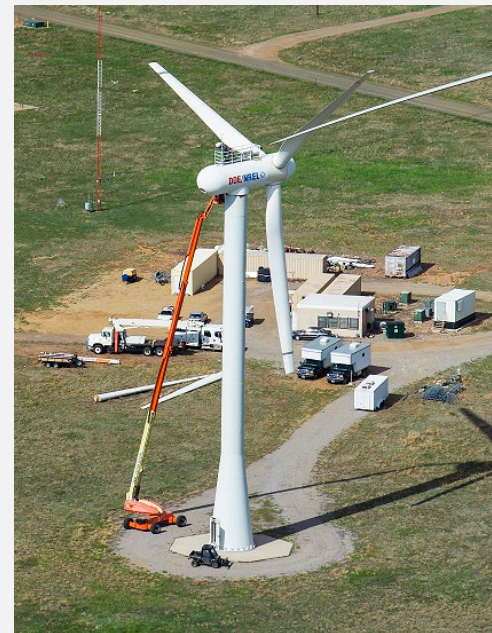
Photo by Dennis Schroeder, NREL 26641
