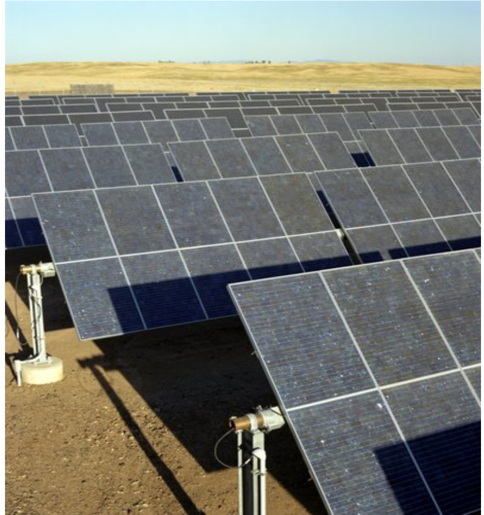
Photo by Warren Gretz, NREL
