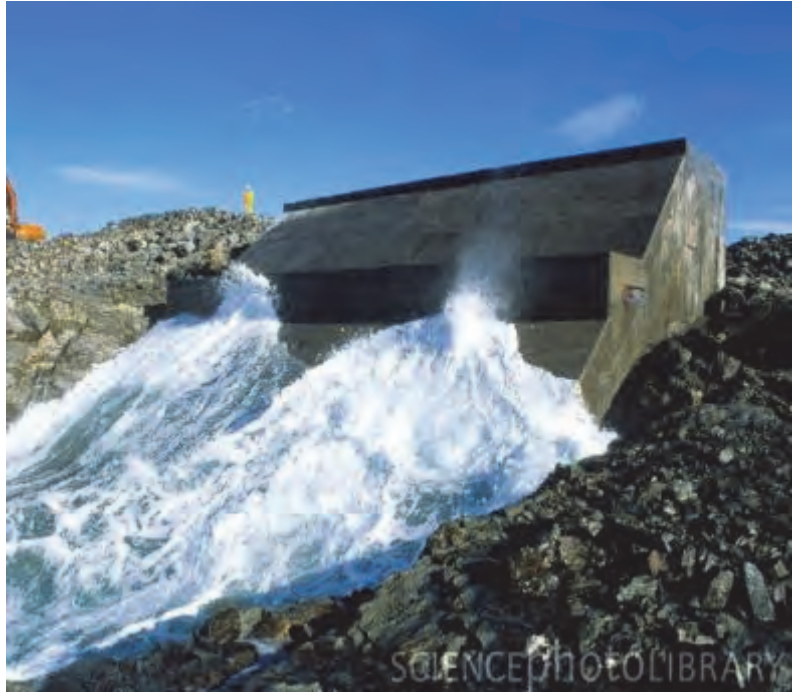
Figure 2-29. The Limpet Wave Power Station in the Isle of Islay, Scotland (Credit: Martin Bond/Science Photo Library)
