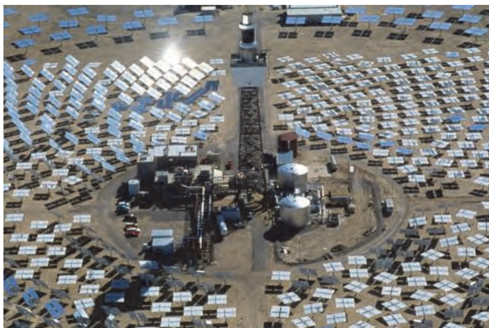
Figure 2-40. Operating Solar Power Facility in Spain
