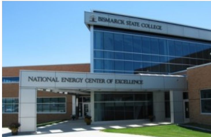
BSC National Energy Center of Excellence
