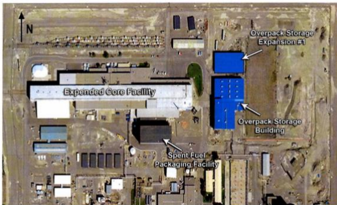
Figure 1: Current ECF and Major Spent Fuel Handling Support Facilities at NRF
