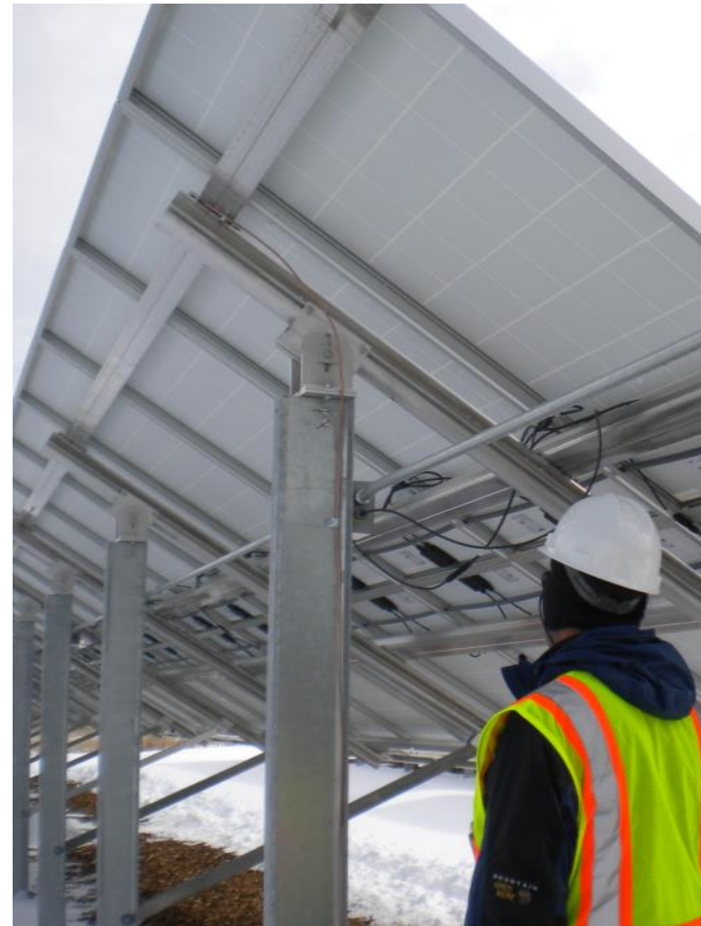
Inspection of a 67-kW PV system at Mesa Verde National Park. Photo by Andy Walker, NREL
