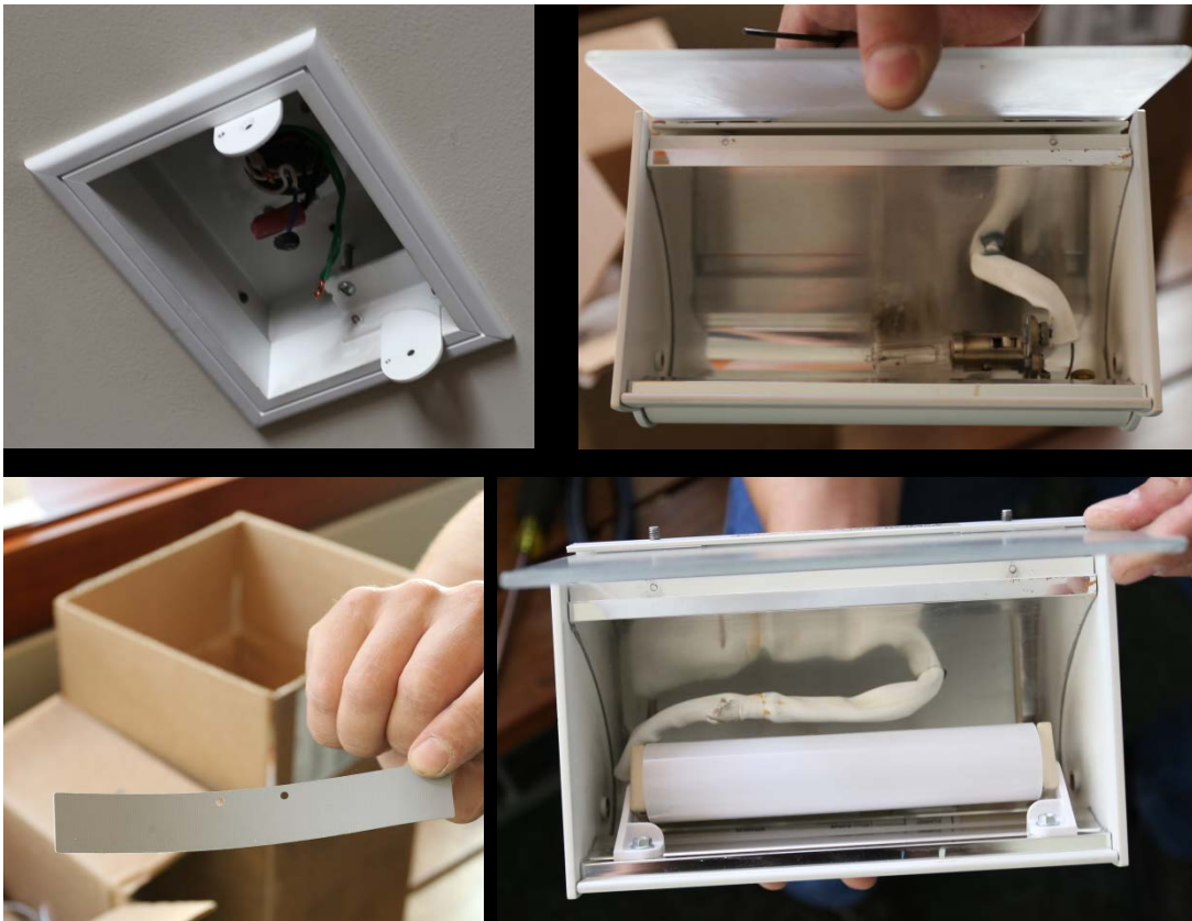
Figure 5. Retrofit of Small Wall Washer from Halogen to LED Module. The trim and mounting frame remained in the ceiling (top left), and the adjustable luminaire housing was removed (top right) so the halogen lamp and socket could be replaced with the LED module (bottom right). A thermal pad (bottom left) was to be attached to the module.
