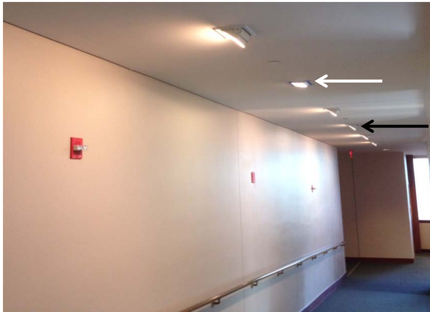
Figure 6. Initial Mock-up of the LED Wall Washer (white arrow) and the 6 in. LED Module (black arrow) with the Existing Halogen Wall Washers (no arrow). The dimming level was 30%. The LED wall washer did not provide light near the top of the wall, or distribute the light as widely on the wall, when compared to the halogen and LED module wall washers.
