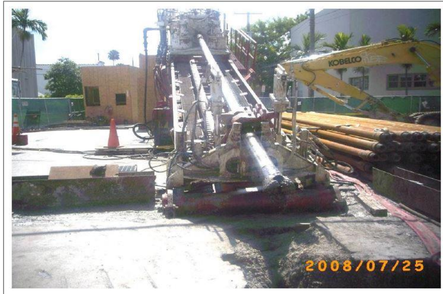
Figure 2-3. Underground Cable Installation – Horizontal Directional Drilling Equipment
