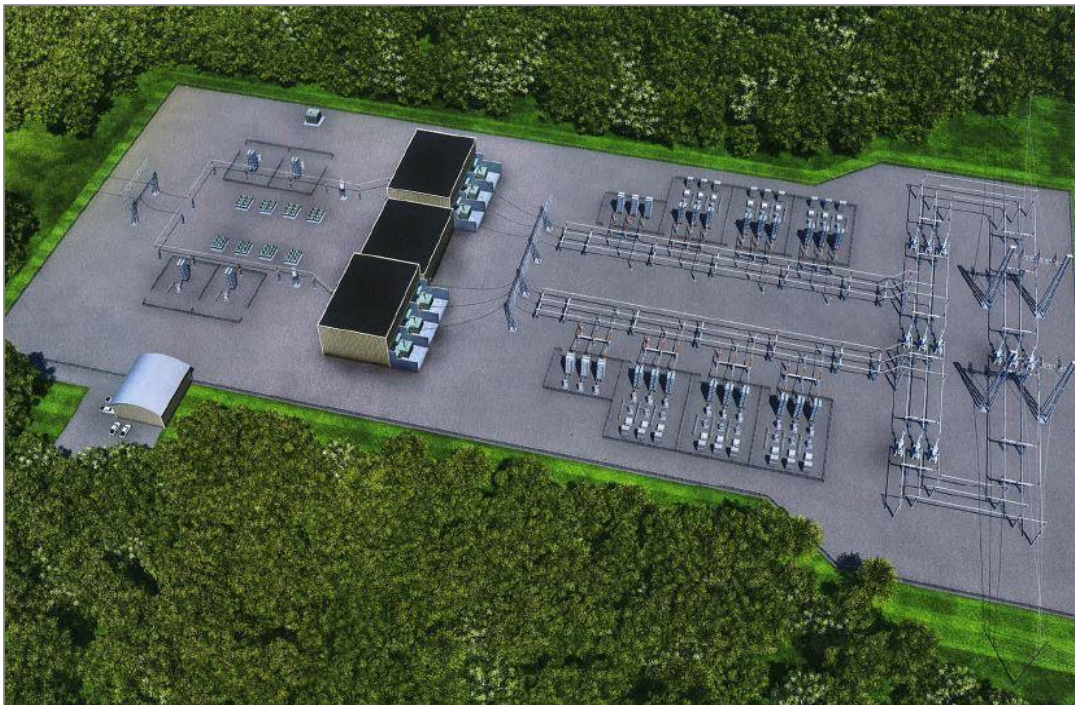
Figure 2-6. Typical Converter Station Layout
