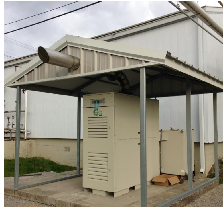
C65 micro-turbine test at ORNL
