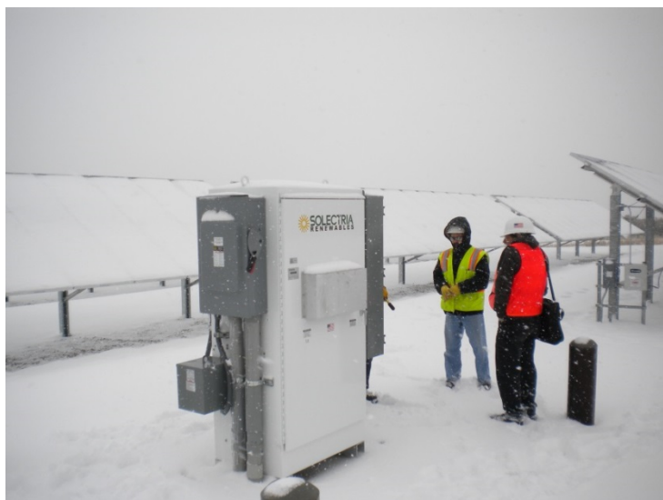
Inspection of a PV system at Mesa Verde National Park. Photo by Andy Walker, NREL
