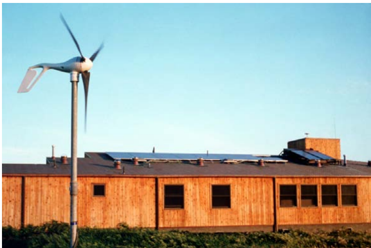
Facility Scale Hybrid System, NPS Range Station, San Miguel Island, CA. Photo by Kent Bullard, NREL 6325496
