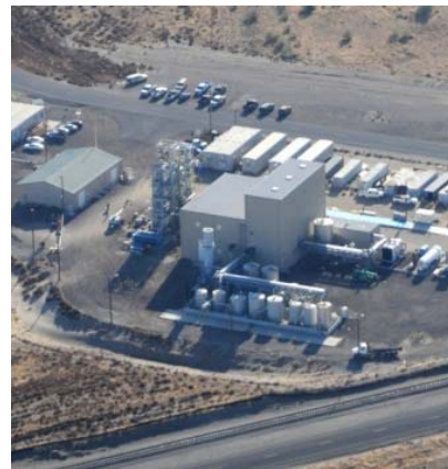
250K GPY IBR Facility Boardman, OR
