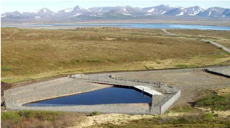
Wastewater lagoon Goodnews Bay Photo Source: ANTHC
