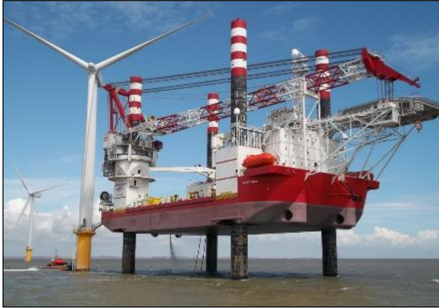
Figure 4. Typical heavy jackup vessel used for offshore wind turbine installations
