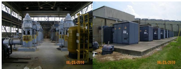
Fig.13. X-630-1 Pump Room and transformer platform.
