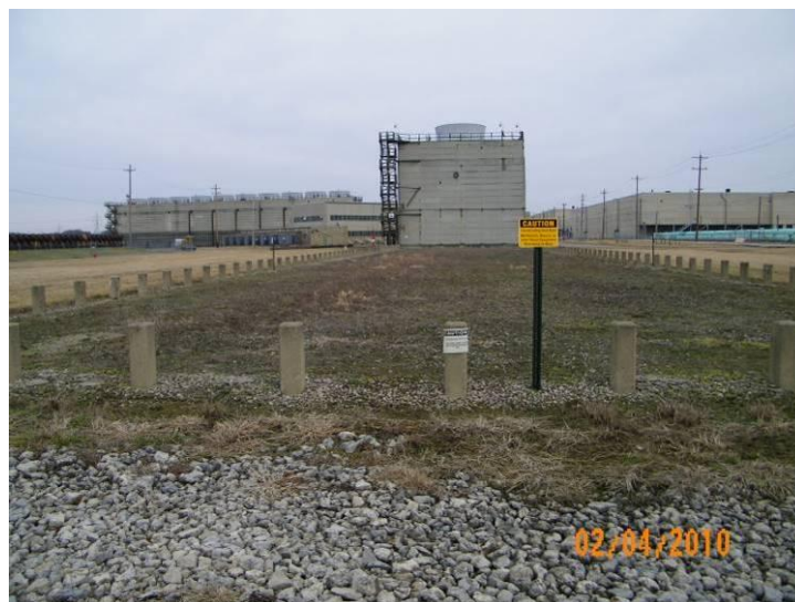
Fig.15. Extended portion of cooling tower basin with concrete slab.
