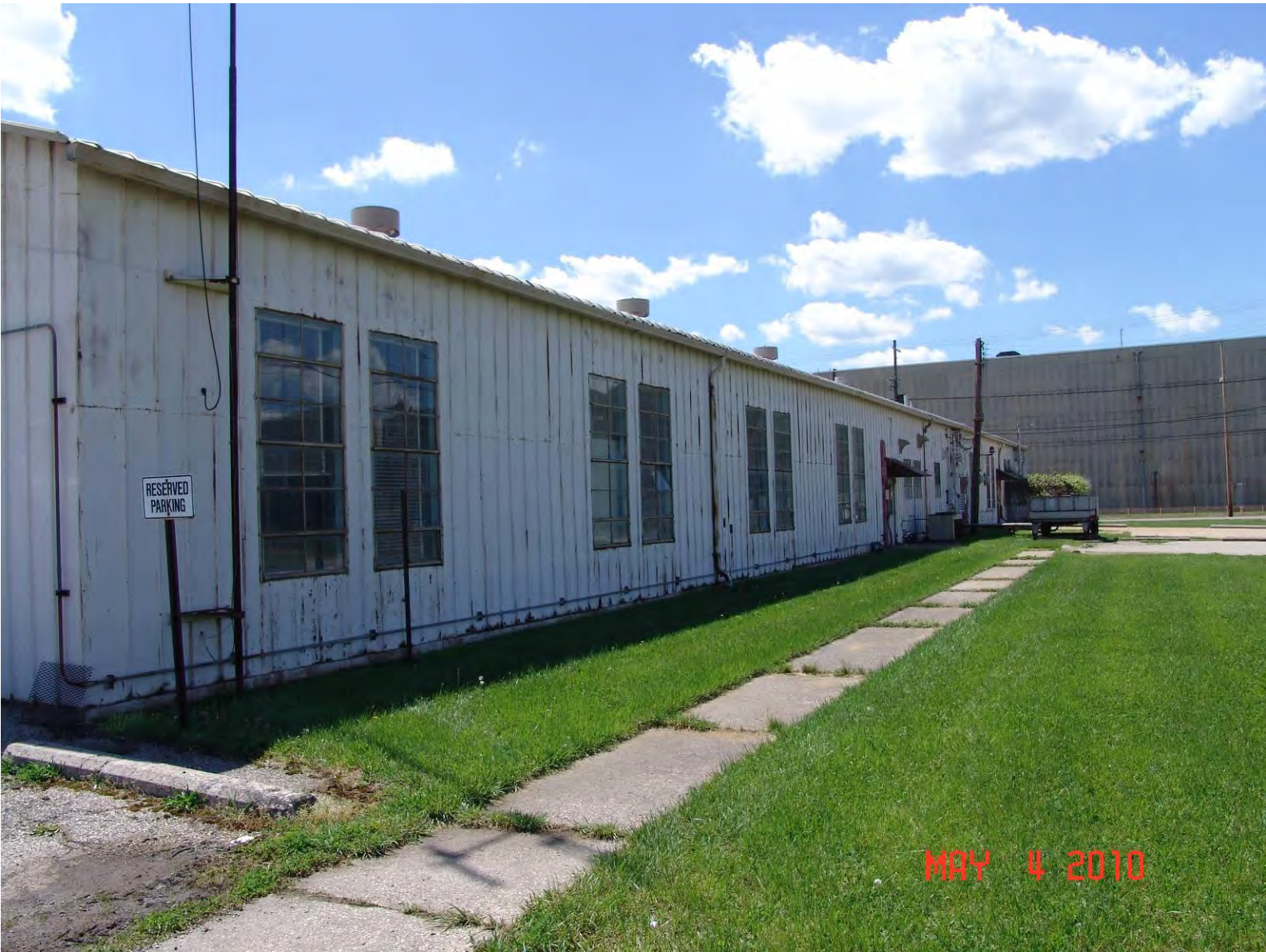
Figure A.3. Building X-103 - exterior (side view) of building.
