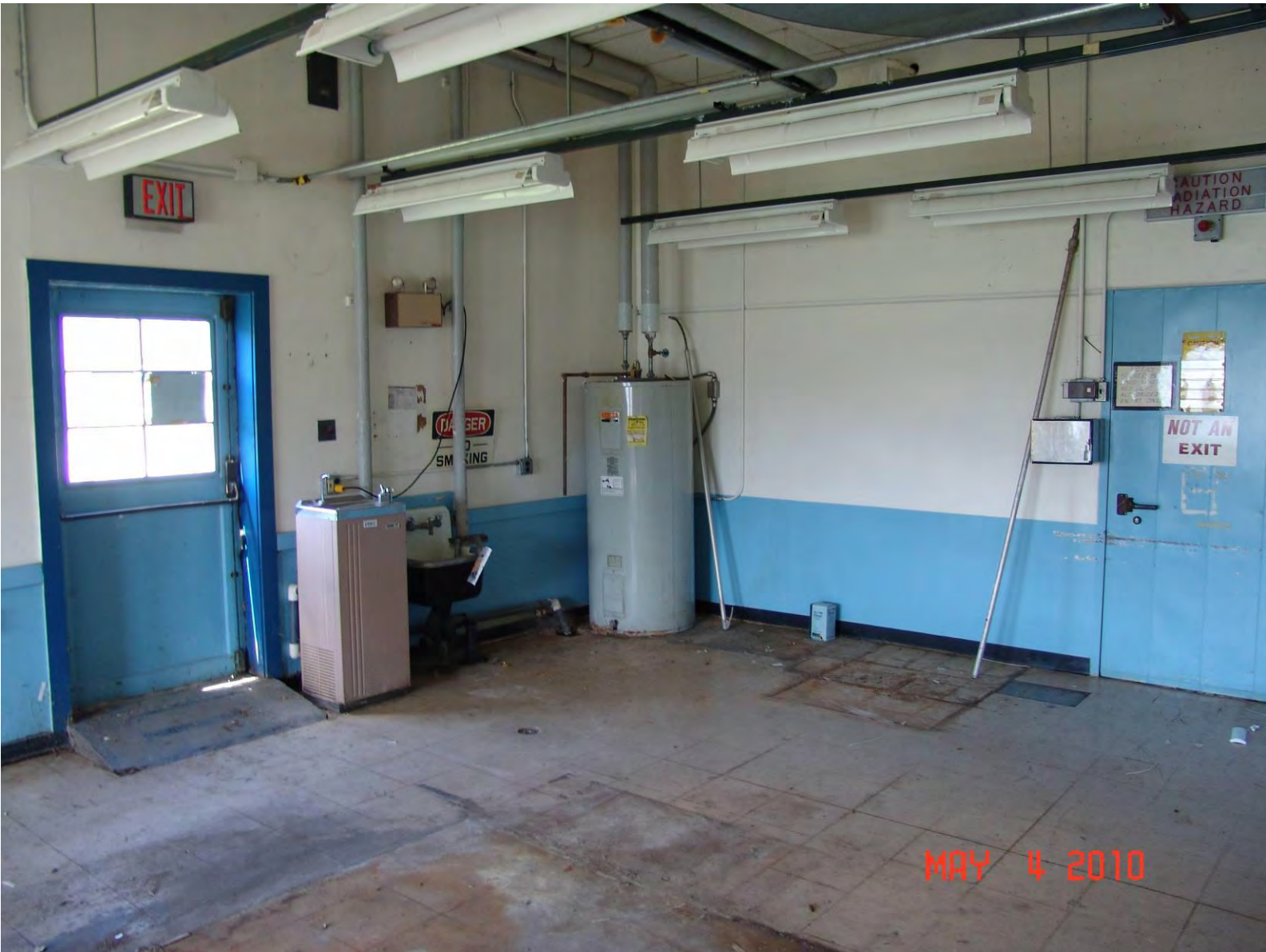
Figure A.2. Building X-103 - representative area showing floor tiles.
