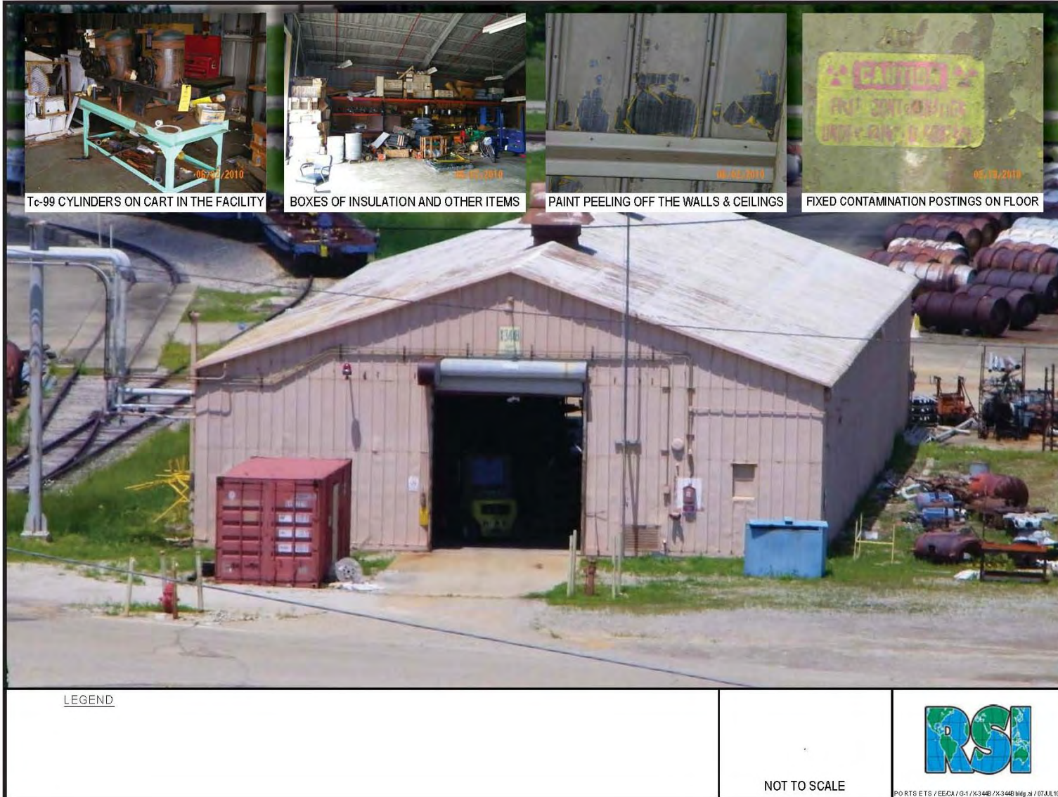
Fig. 9. Building X-344B exterior with insets of building interior.
