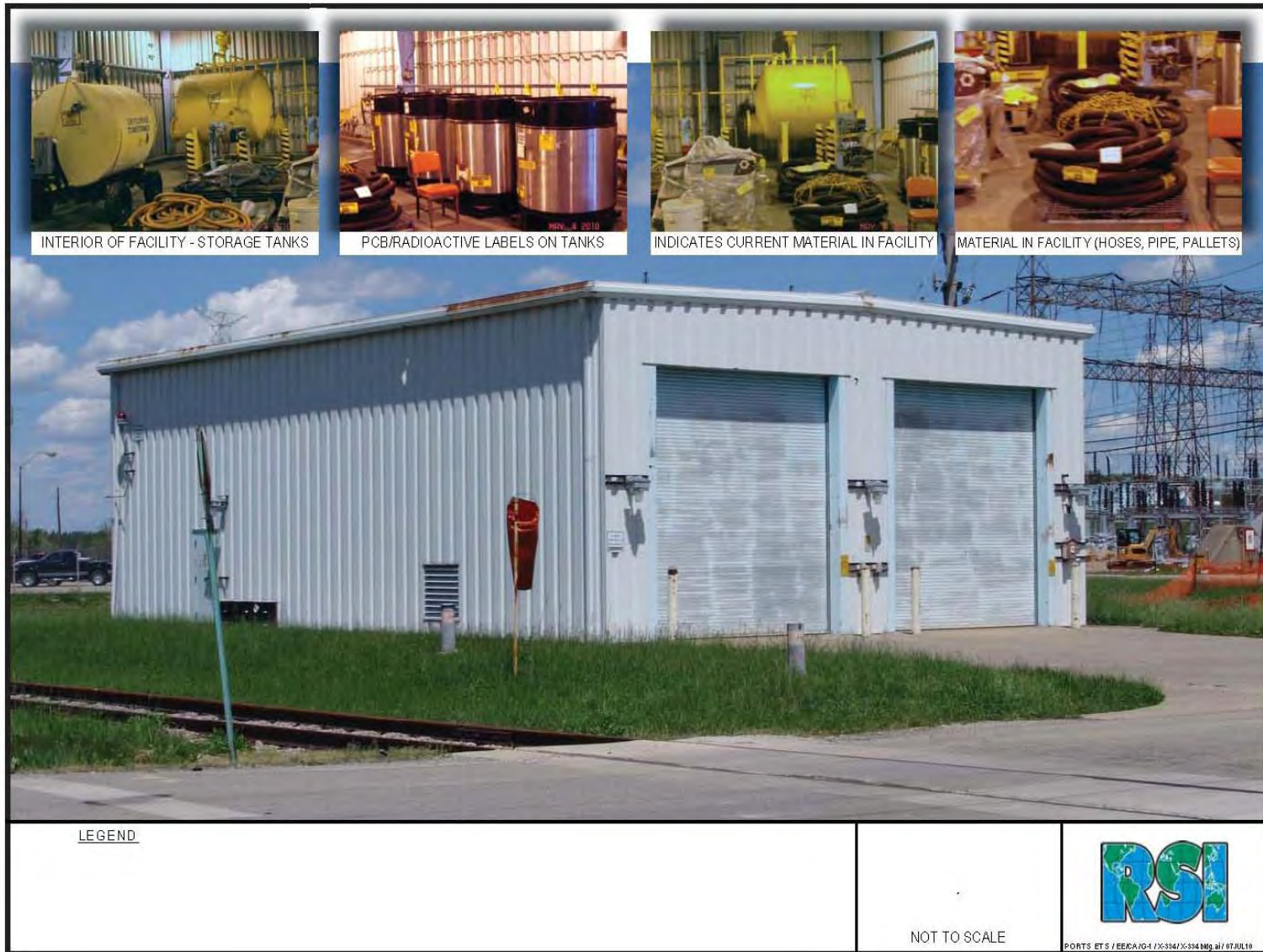
Fig. 6. Building X-334 exterior with inserts of building interior (photo taken May 2010).
