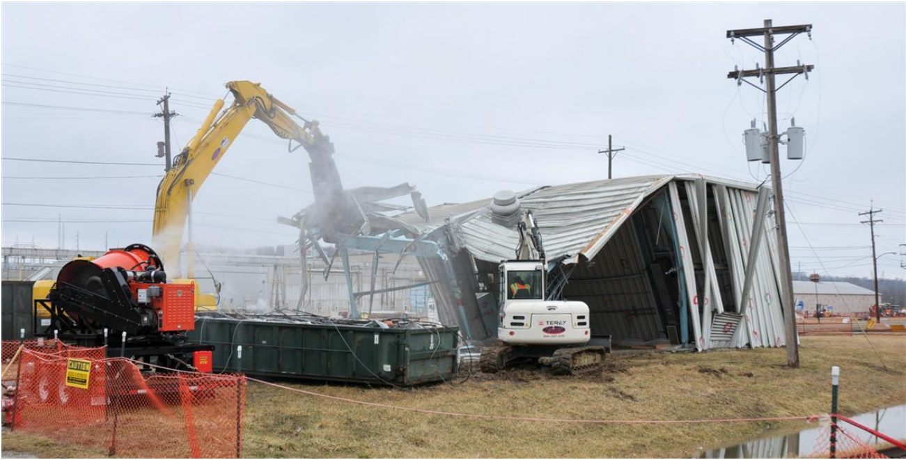
Photo 6. X-334 Building demolition
