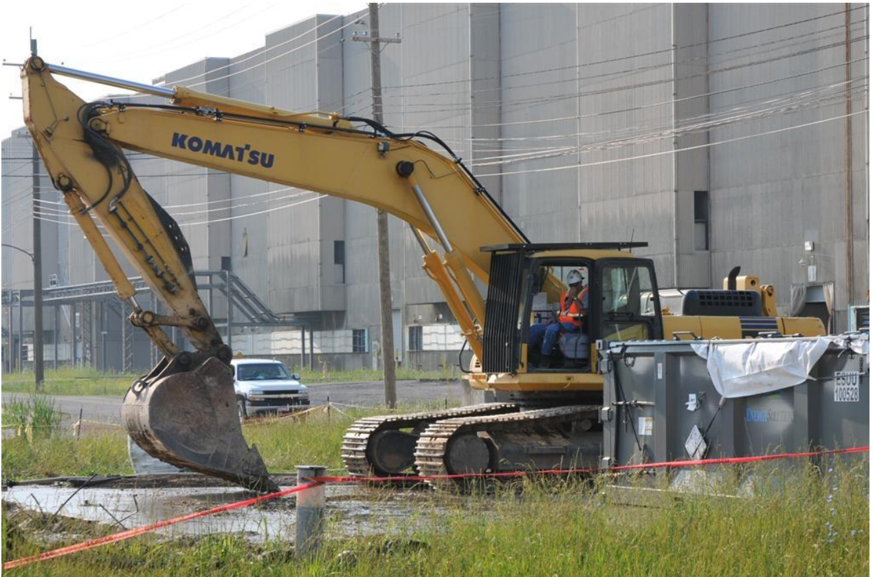
Photo 8. Slab removal
