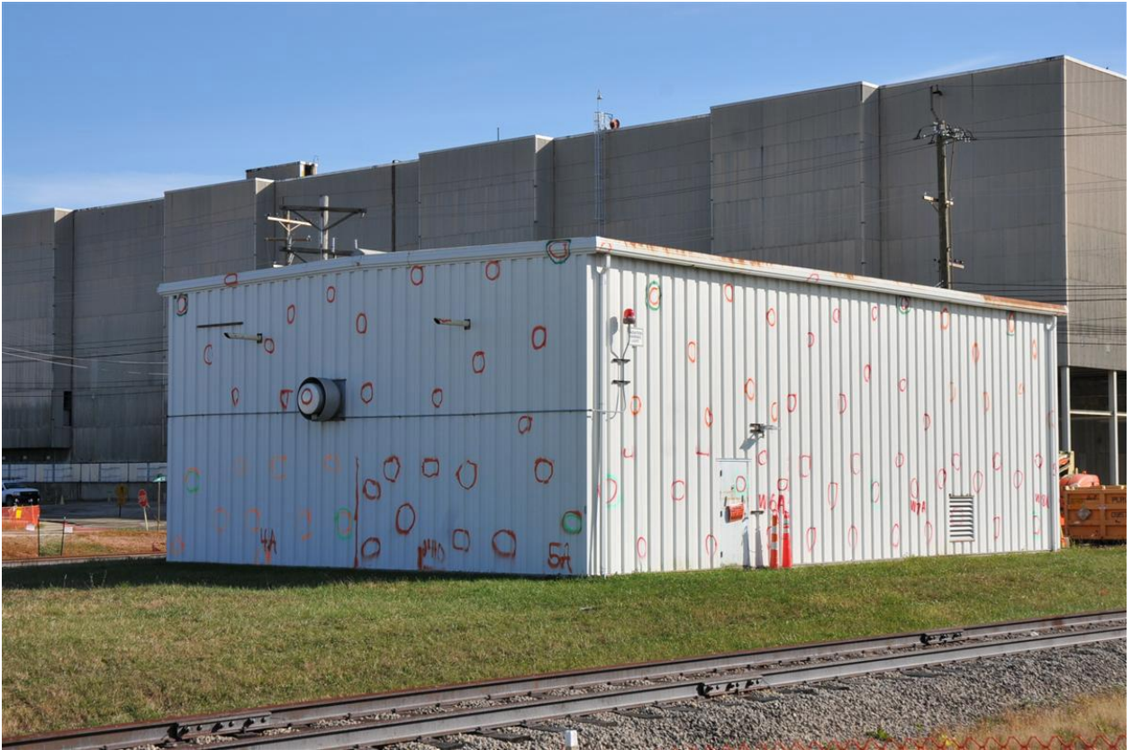
Photo 3. Rear and west side of the X-334 Building facing southeast
