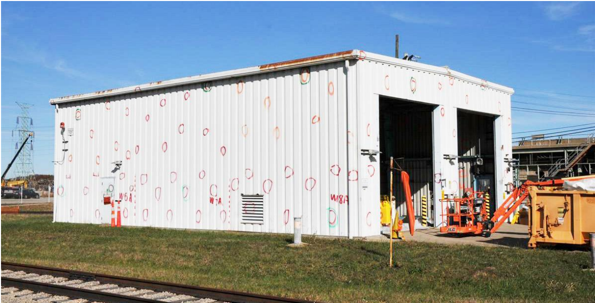
Photo 1. X-334 Building facing northeast
