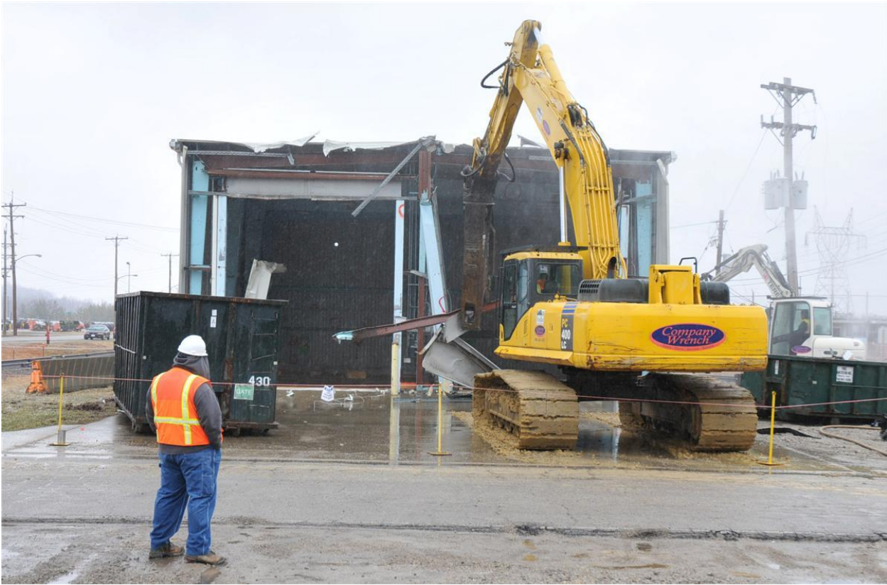
Photo 5. X-334 Building demolition
