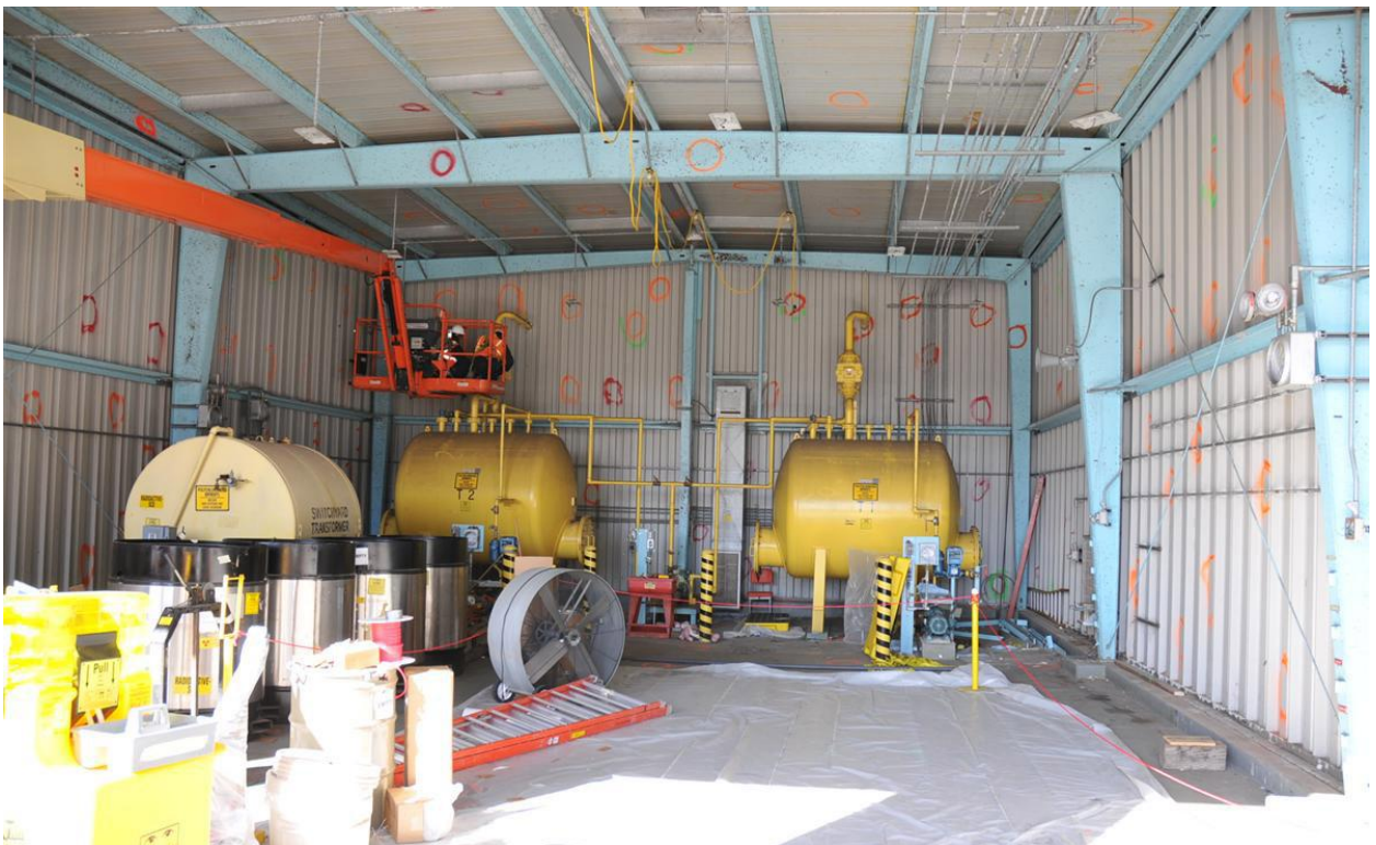
Photo 4. Interior of the X-334 Building
