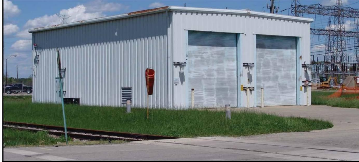
Figure 3. Photograph of X-334 Building before demolition, facing northeast
