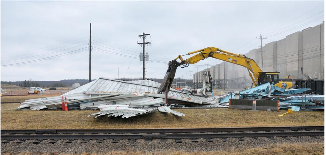
Photo 7. X-334 Building demolition
