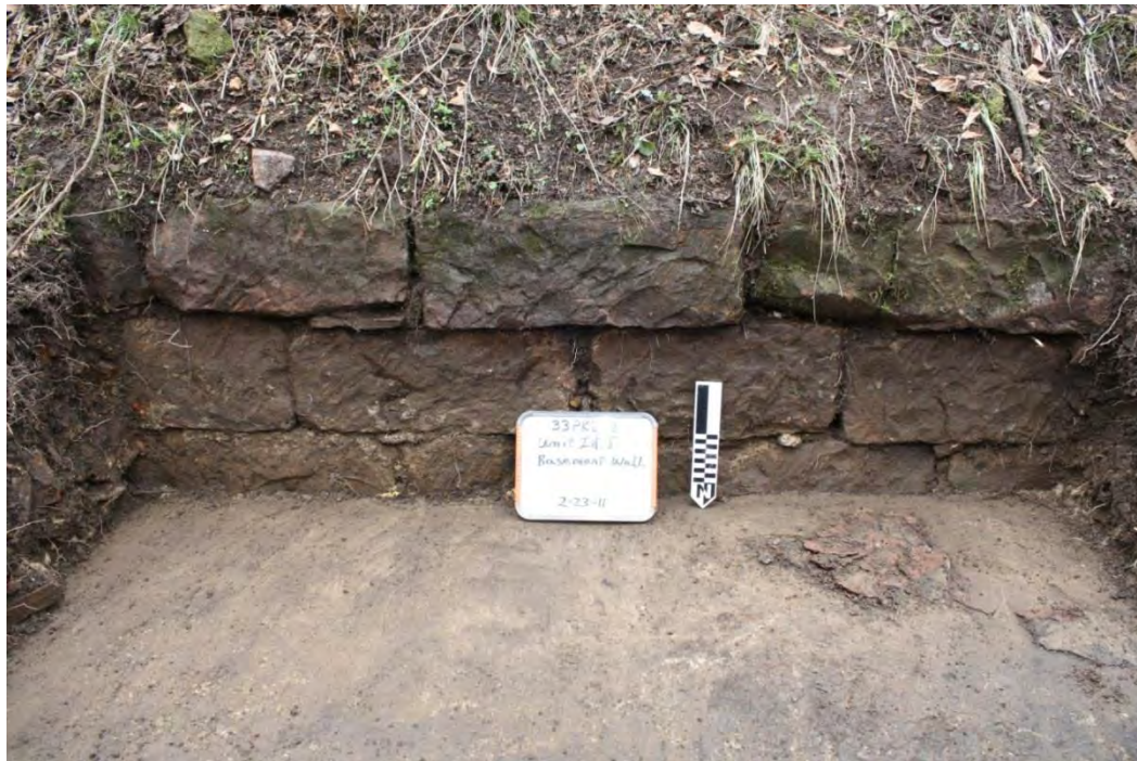
Figure 69. Photograph of a cut stone masonry cellar foundation wall (with a poured concrete floor) at Ruby Hollow Farmstead (33Pk203).
