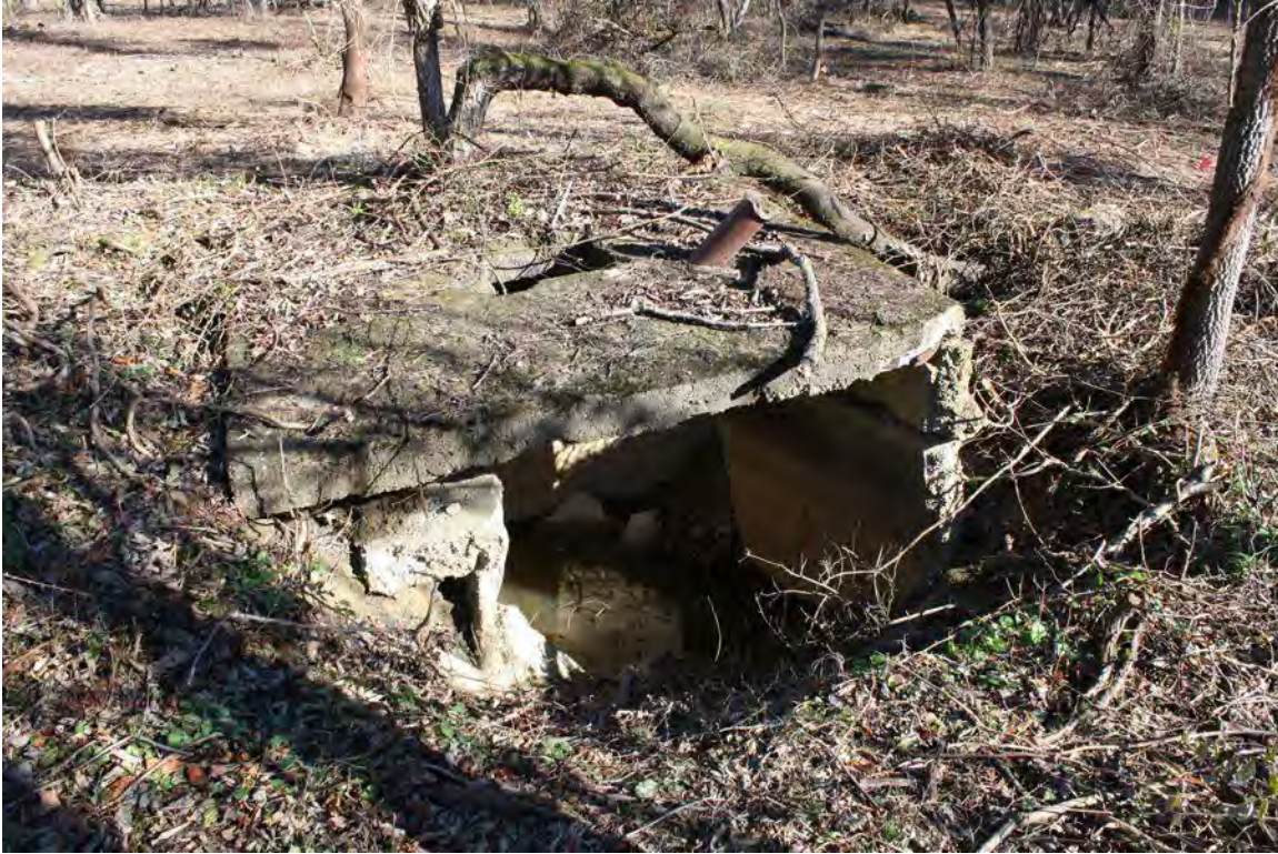
Figure 100. Photograph of the poured concrete cistern at Mechling Farmstead (33Pk318).
