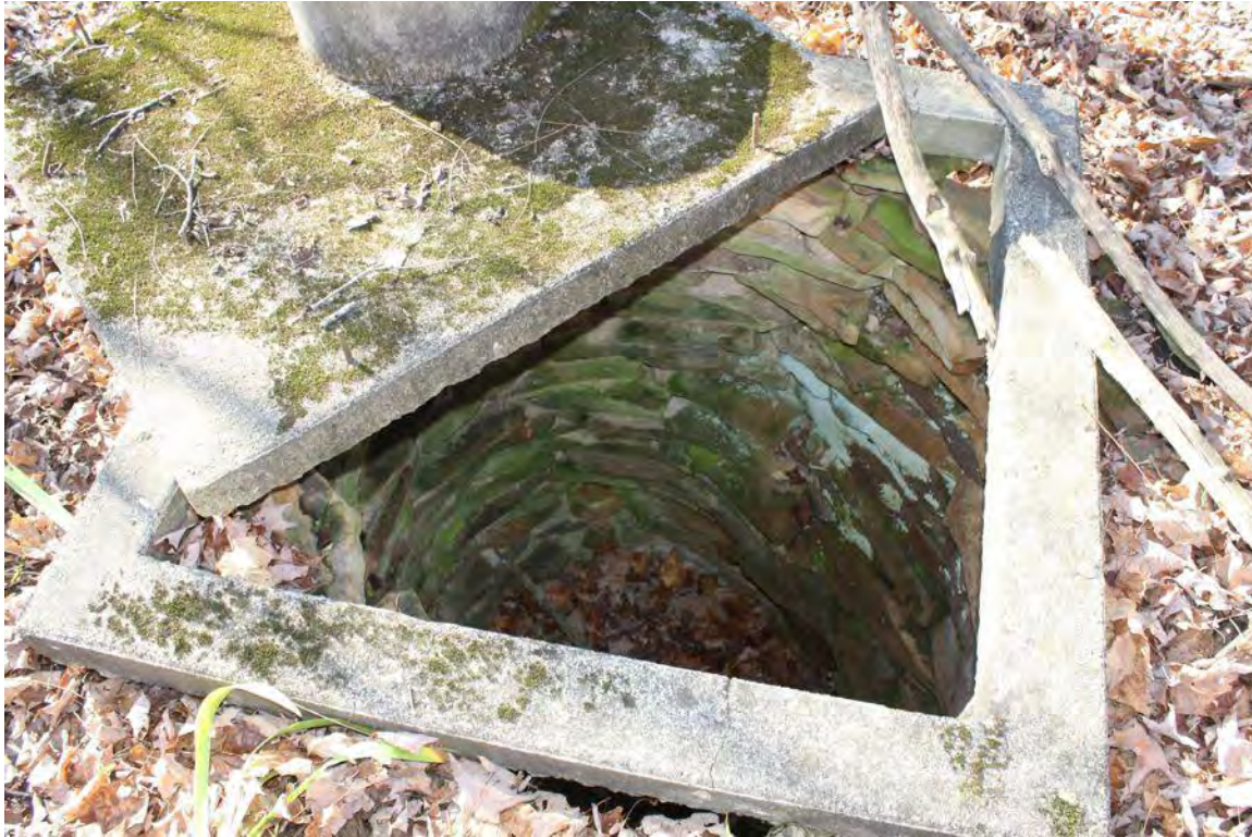
Figure 97. Photograph of the septic system at Brodess Farmstead (33Pk311).
