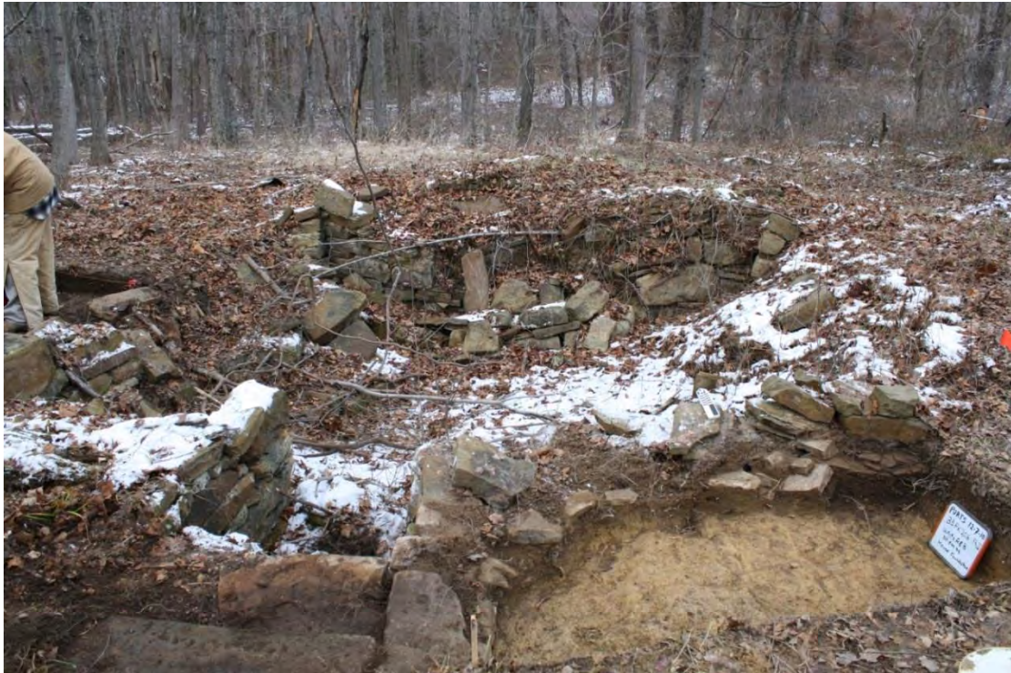
Figure 68. Photograph of a rough fieldstone masonry cellar foundation (partially collapsed) at Terrace Farmstead (33Pk206).
