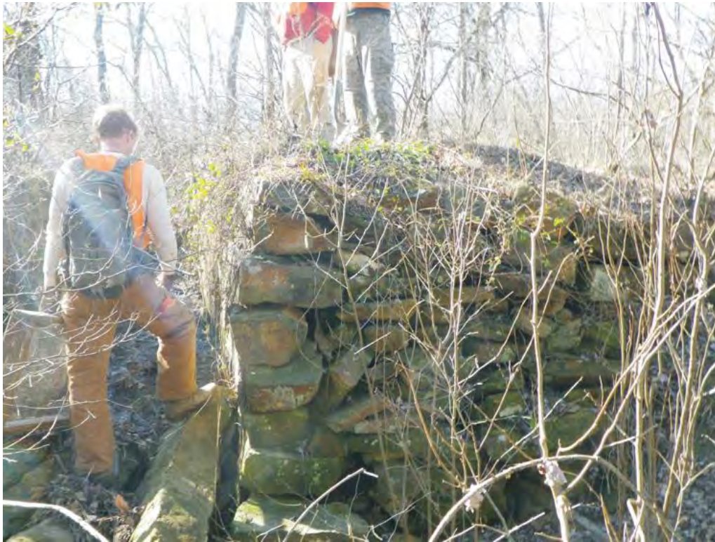
Figure 52. Photograph of the 33Pk363 bridge abutment (from Garrard and Burden 2012).
