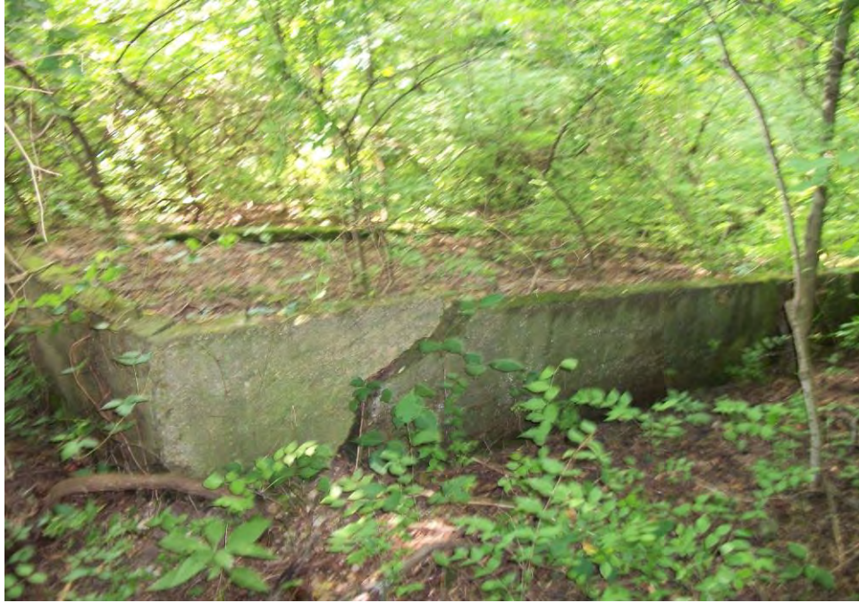
Plate 29. Building 3 at 33PK324/HMBL 50; facing west-northwest.
