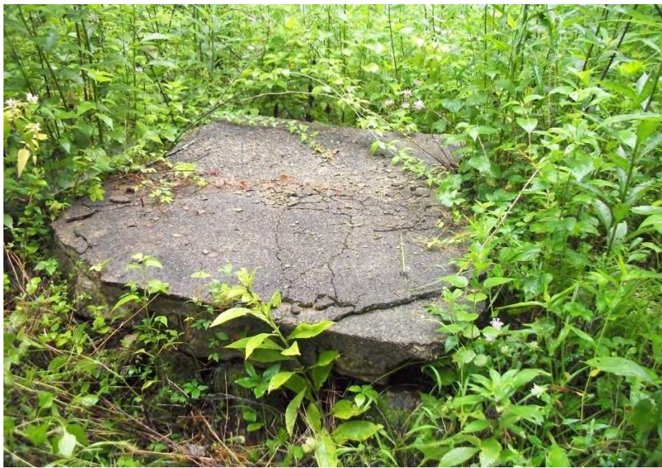
Plate 10. Concrete stoop or capped well at 33PK322/HMBL 4; facing northeast.
