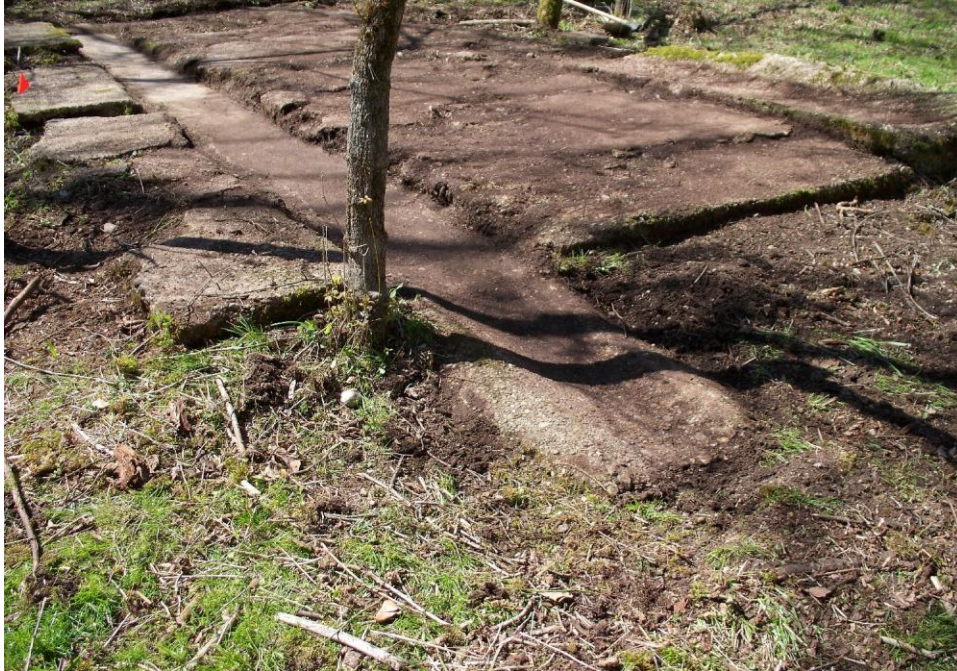
Plate 7. View facing northwest showing the concrete feed and slop floor at Building 3, a barn, at 33PK212. The down slope discharge of the slop trough is visible in the center foreground.
