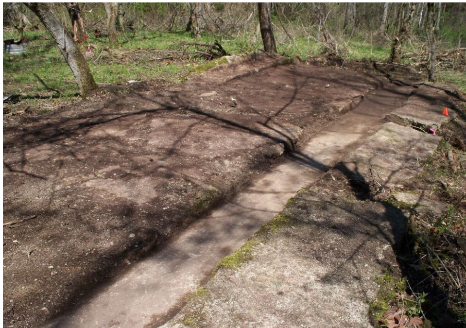
Plate 6. View facing northeast showing the concrete feed and slop floor at Building 3, a barn, at 33PK212.
