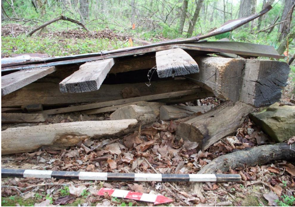
Plate 19. Detail view of the roof construction at 33PK213, facing west.
