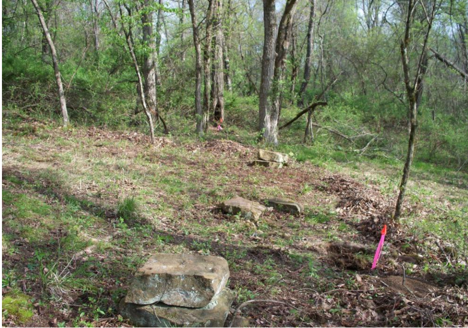
Plate 21. View facing northwest of three of the support piers for the barn at 33PK213.
