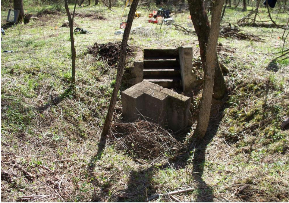
Plate 1. View facing northeast showing Building 1 at 33PK212.
