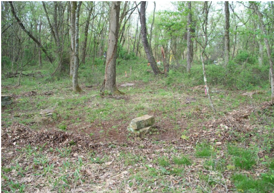
Plate 22. View facing south of the six support piers for the barn at 33PK213.
