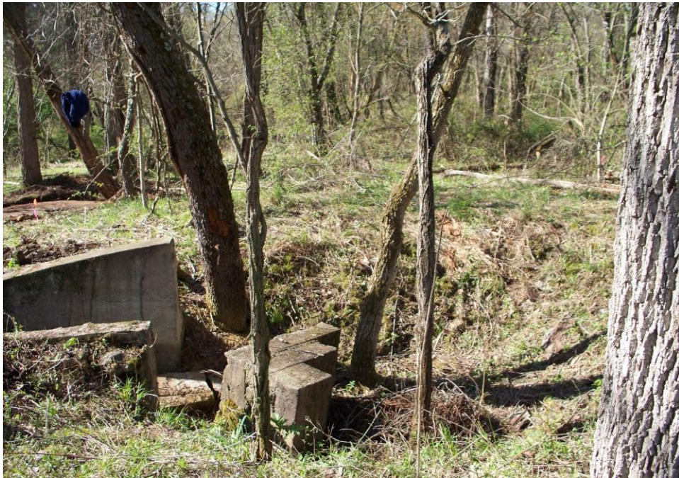
Plate 2. View facing south showing Building 1 at 33PK212.
