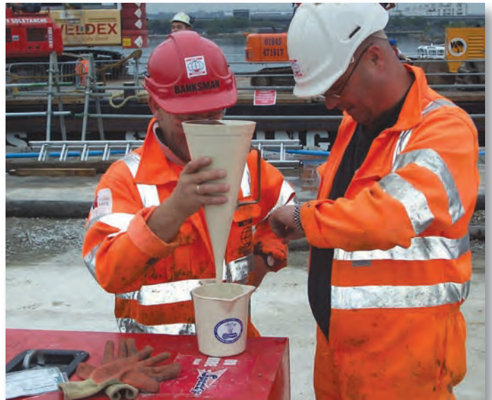
Slurry technicians are available for on-site technical support and training.
