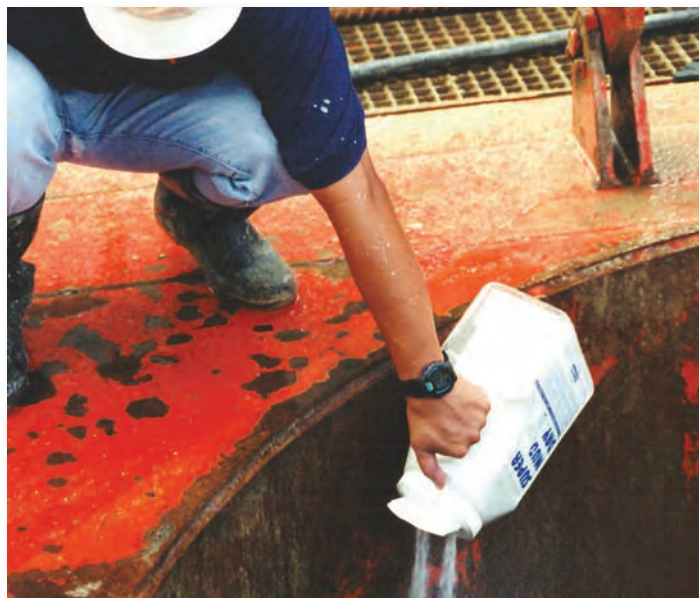
Mixing Directly into the Excavation
