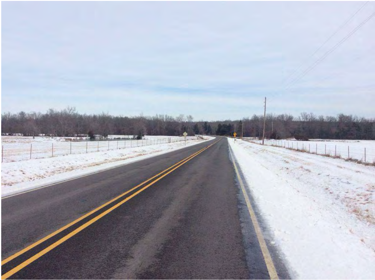
View south toward PR along scenic highway. View includes scattered trees, dense forest, roadway, open grassy area, wood power poles, and fences.
