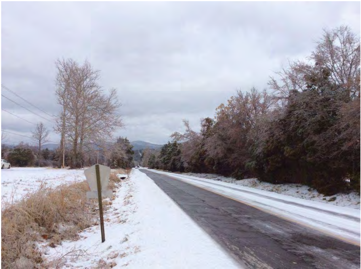
View north along the Route 21 Scenic Byway. The area is very rural with only a few single family residences in the vicinity.
