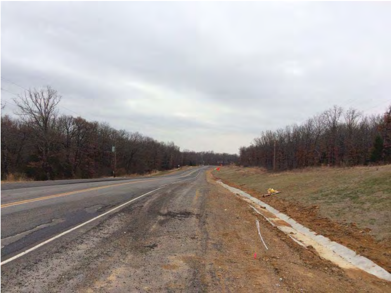
View south of PR crossing the Trail of Tears along SR 100, a scenic byway. View includes roadway, wood pole power lines lining both sides of road, and dense forest on both sides of road.
