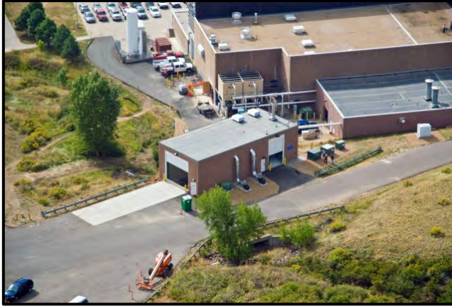
Renewable Fuel Heat Plant
