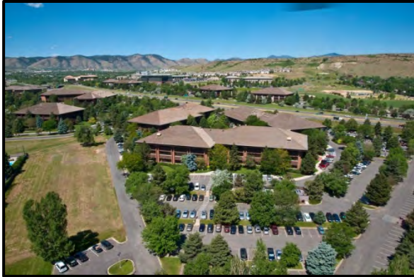
Denver West Office Park
