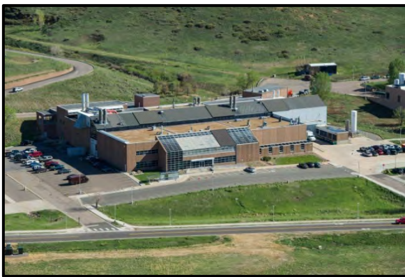
Field Test Laboratory Building
