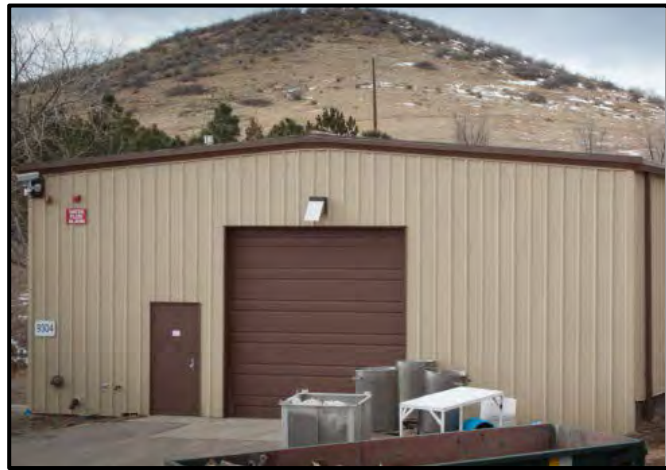
Bulk Storage Building
