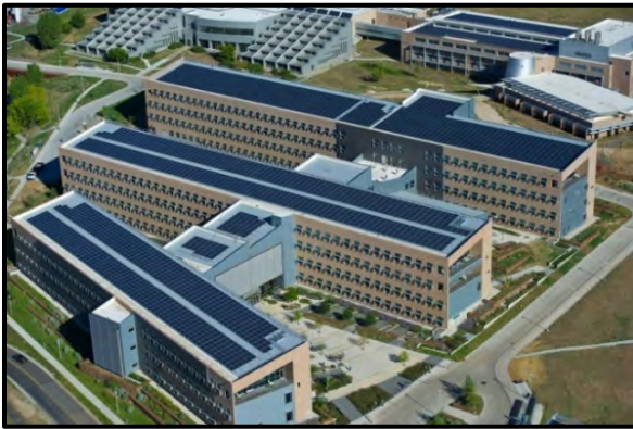
Research Support Facility
