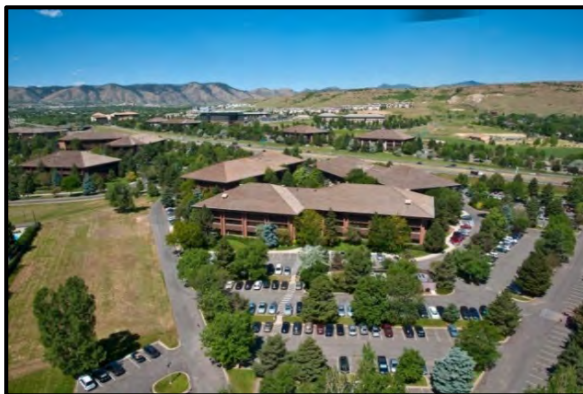
Denver West Office Park
