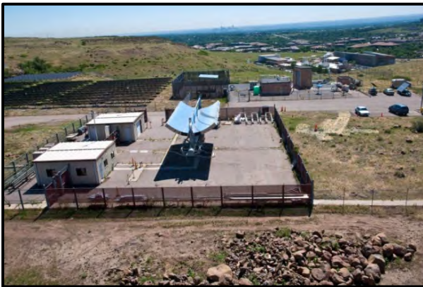
Solar Industrial Mesa Test Area
