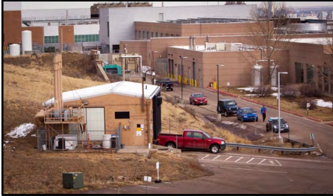
Waste Handling Facility
