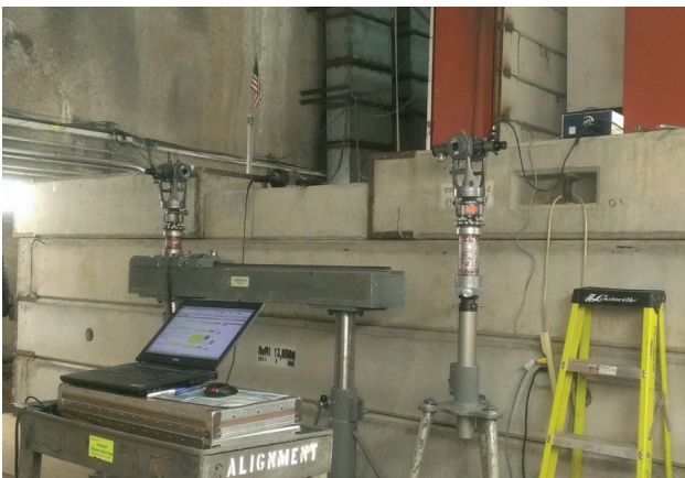
Exhibit 4-9: NuMI Work Cell Shield Wall
