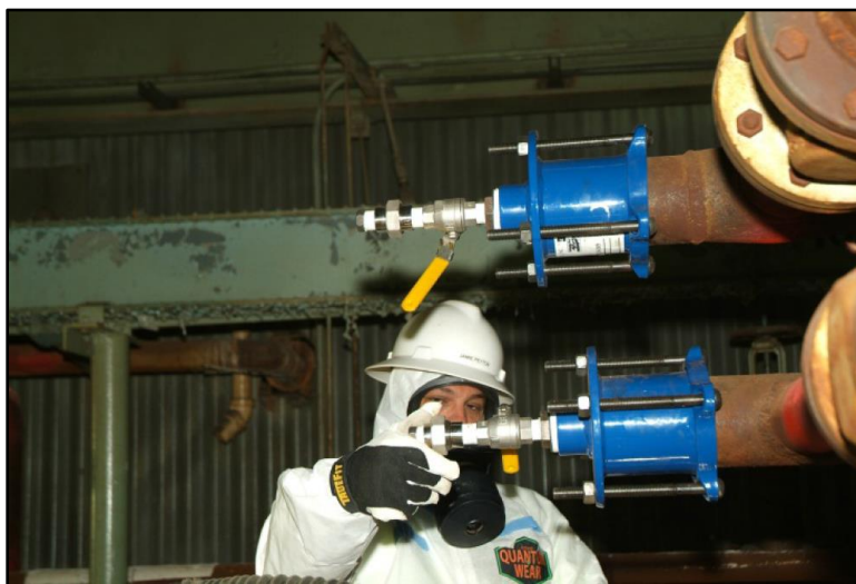
Figure 3.1. Purging UF 6 from Piping in the C-410-Building
