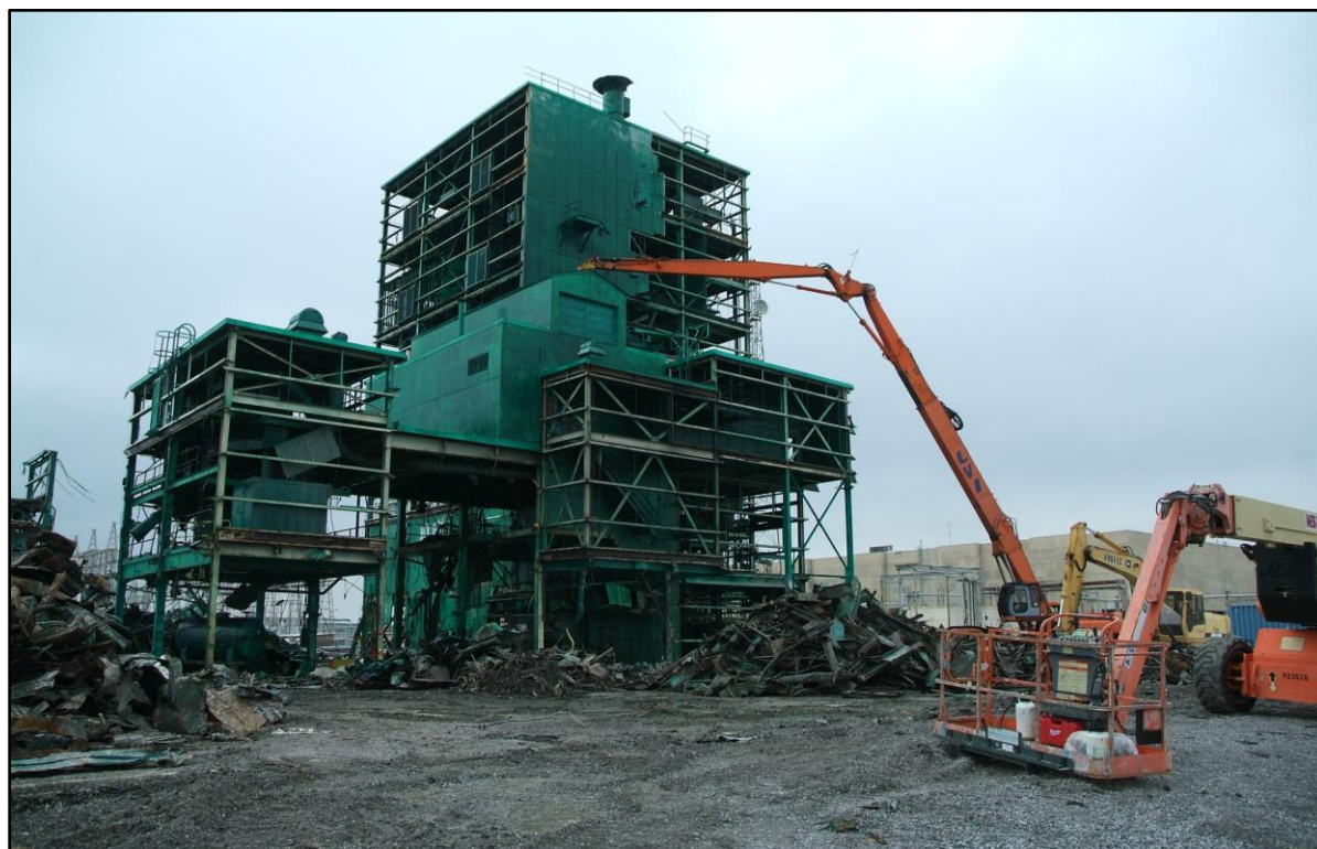
Figure 3.4. C-340 Building Demolition
