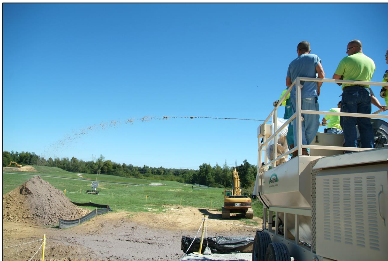
Figure 2.1. Posi-Shell® Application to C-746-U Landfill
