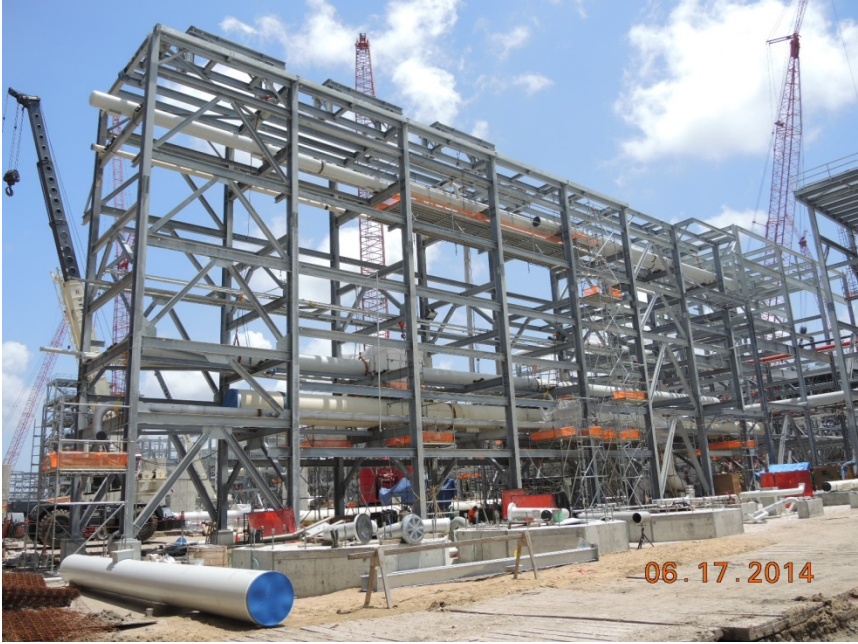
Train 2 installing pipe
