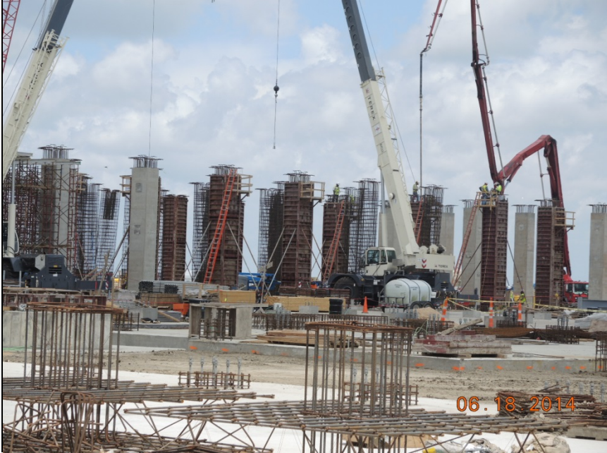
Train 3 pouring concrete ethylene columns
