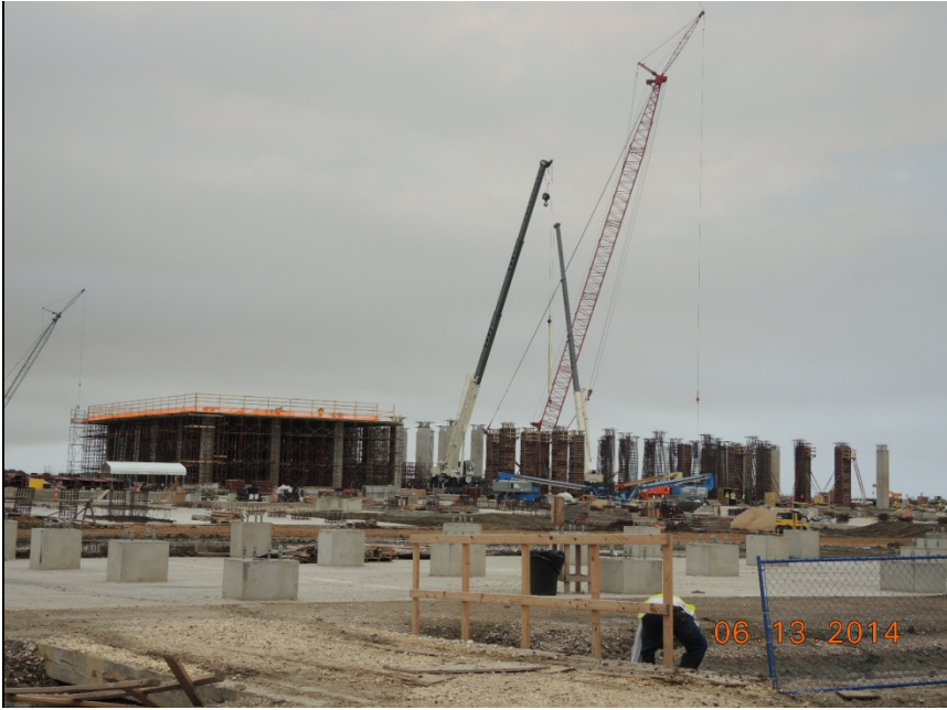
Train 3 tabletop and columns
