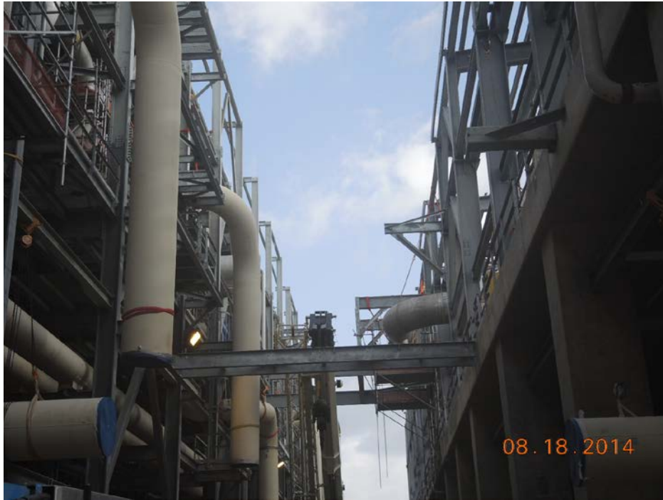
Train 1 Installing Pipe
