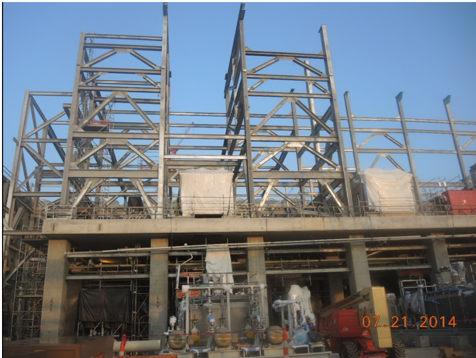
Train 1 Installing Steel on Upper Deck
