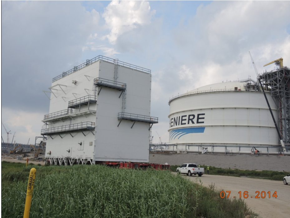
Train 1 Moving the Methane Cold Box to Site
