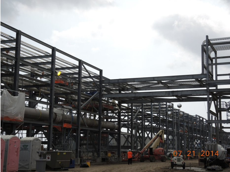
Train 1 & OSBL Installing Cable Tray & Pipe
