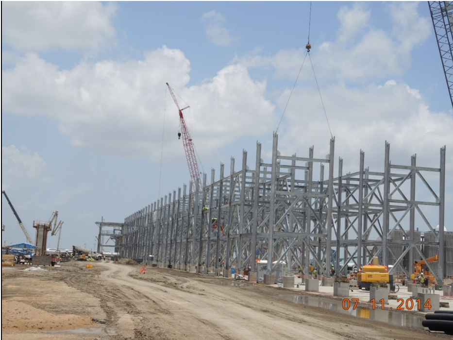
Train 3 Installing Steel
