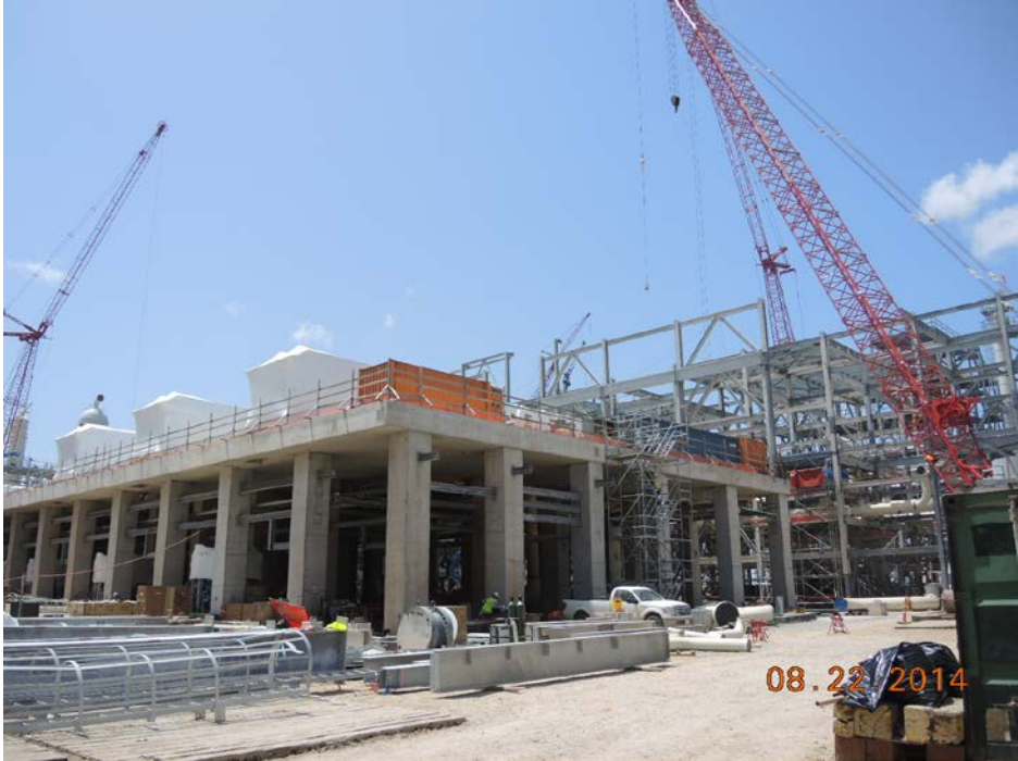
Train 2 Setting of Turbines and Compressors Complete
