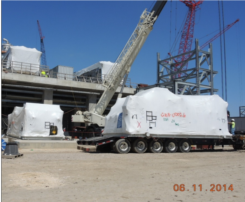
Train 1 installing lube oil skids
