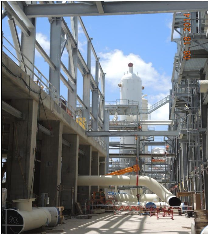
Train 1 installing pipe from under tabletop
