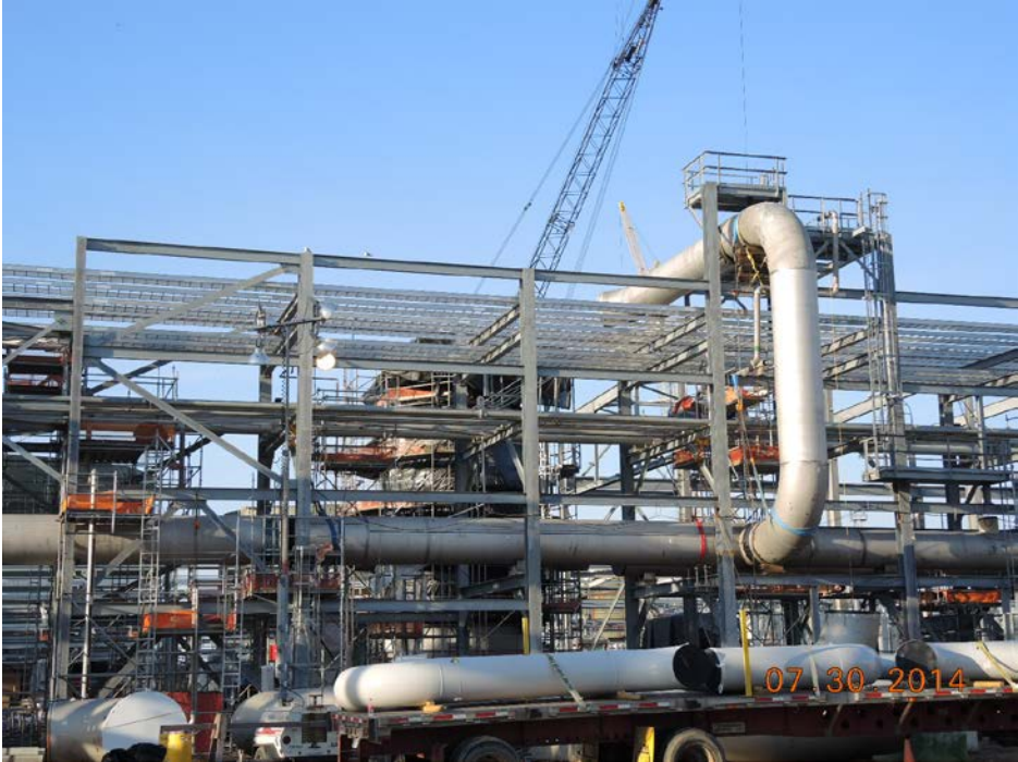
OSBL Stage 1 Installing Pipe and Cable Tray
