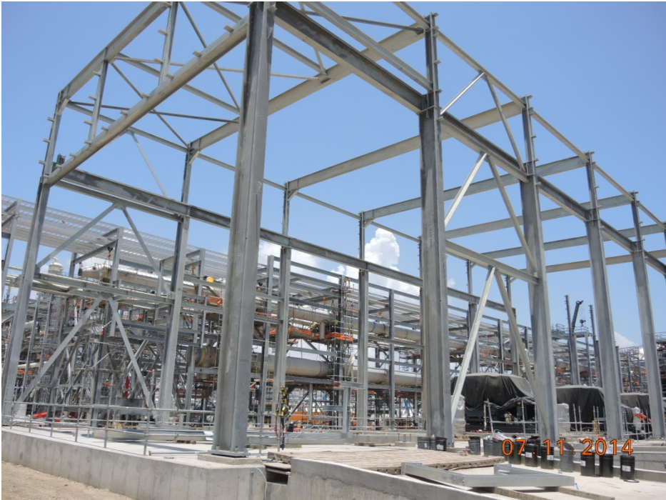
OSBL Installing Steel for the BOG Compressor Building
