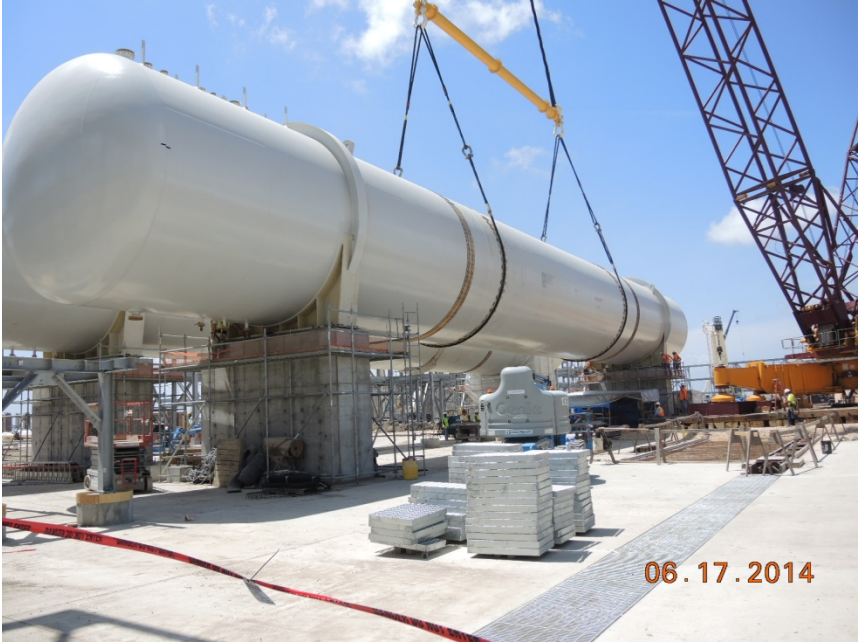
OSBL installing propane storage drum
