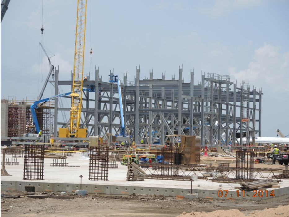
Train 3 Installing Steel
