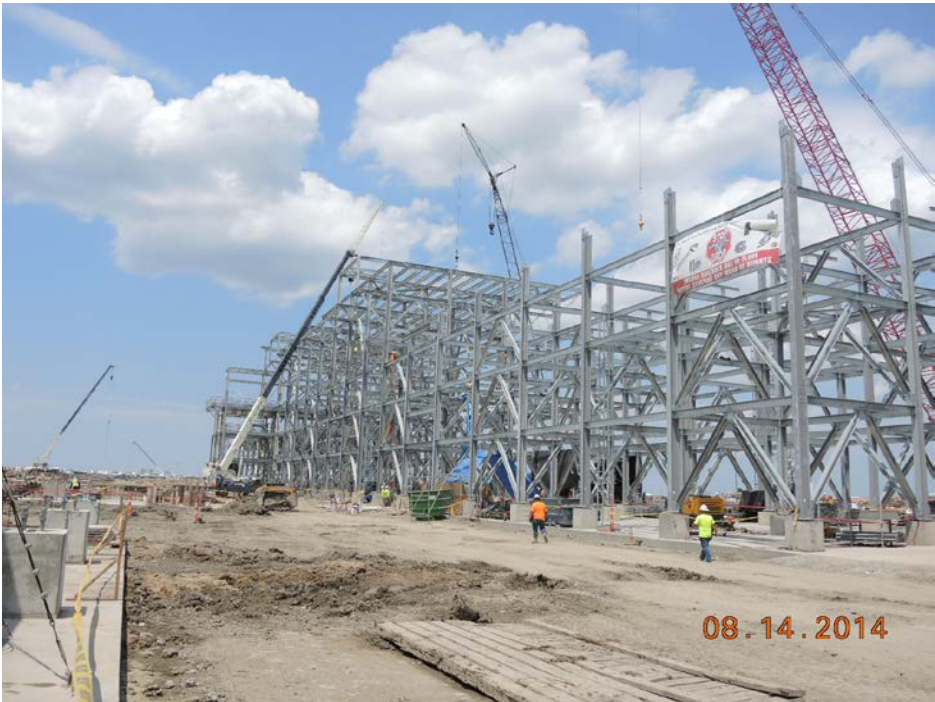
Train 3 Installing Steel on Propane Rack
