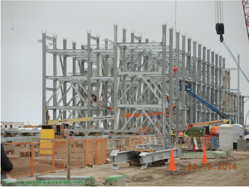
Train 3 installing steel on propane rack
