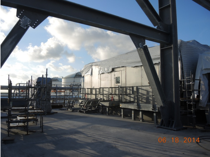
Train 1 installing steel and platform around turbines
