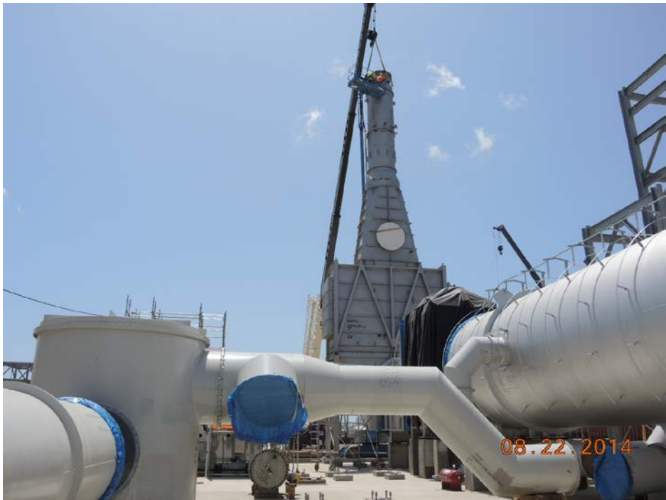
Train 2 Installing Stack on Thermal Oxidizer PreHeater
