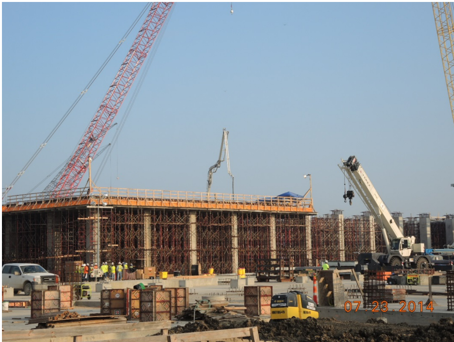
Train 3 Pouring concrete
