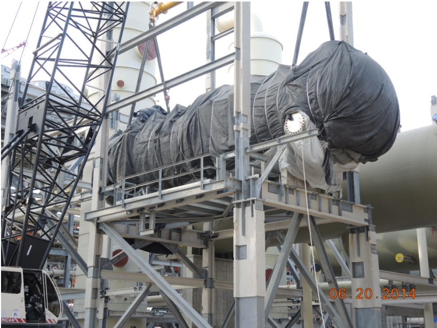
Train 1 installed ethylene surge drum
