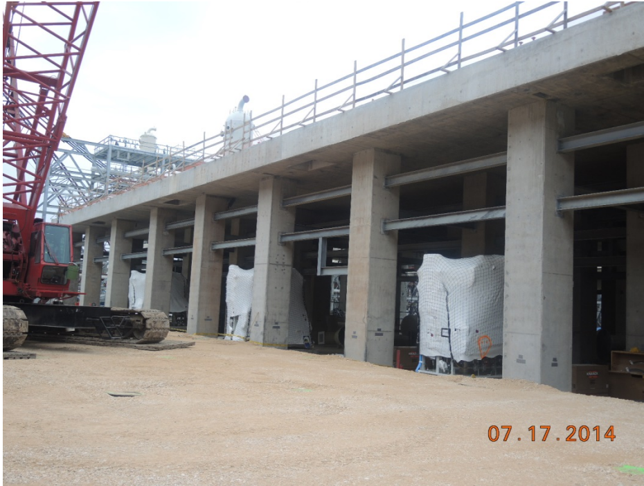
Train 2 Installing Fuel Gas Scrubber Skids
