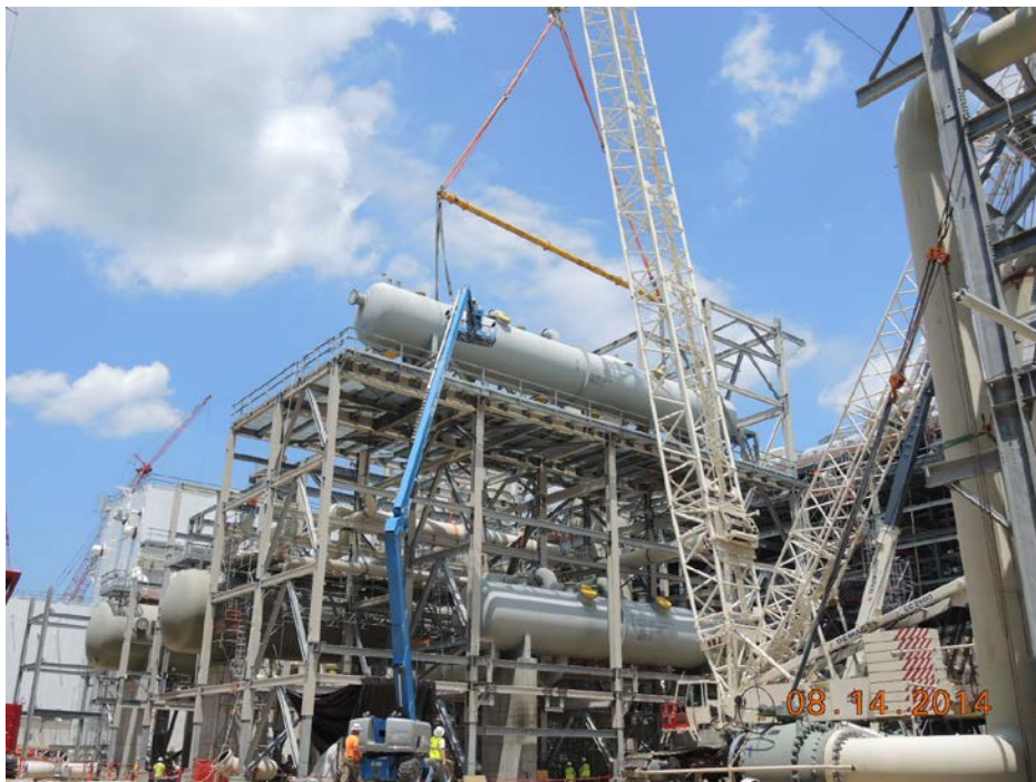
Train 1 Setting IS Propane-Methane/Ethylene Feed Chiller
