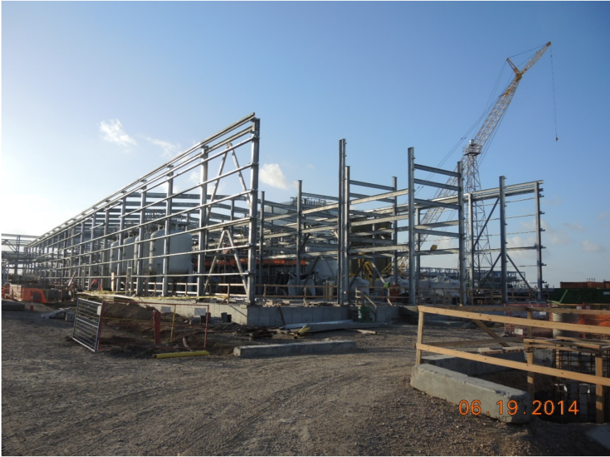
OSBL Erecting Water Treatment Building
