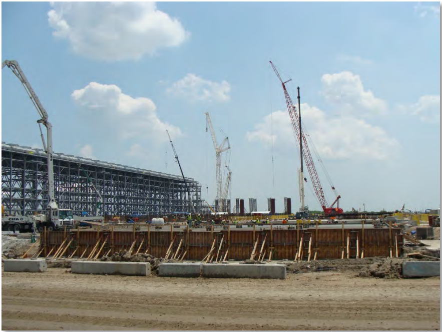
Train 2 132D (cryo air coolers piperack) (16-Aug-2013)
