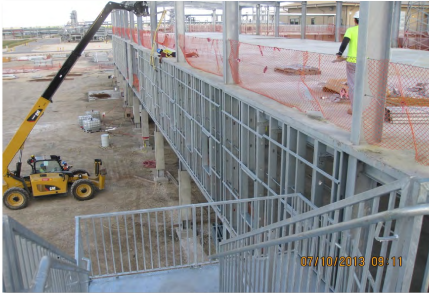
New Operations & Maintenance Building - Exterior Wall Panel Installation (10-July-2013)
