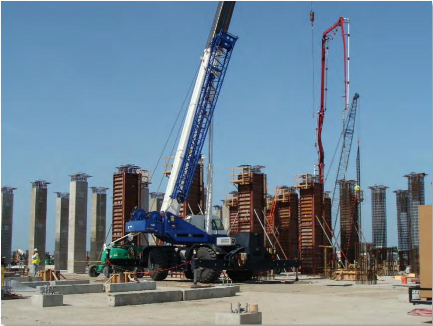
Train 1 area 132A01 (compressor columns) (29-July-2013)
