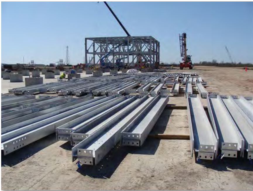
Steel Erection and Staging, Area 131N (8-Mar-2013)
