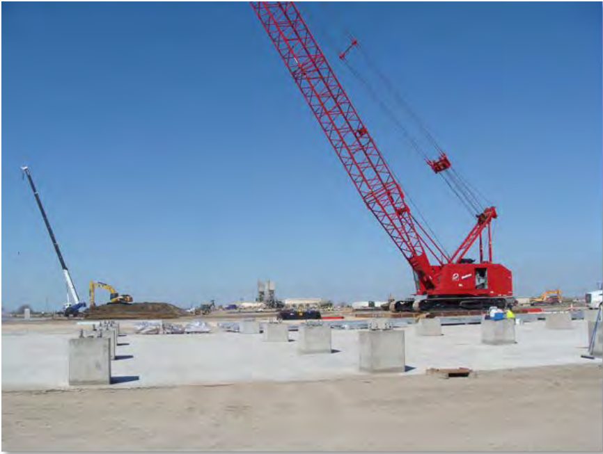
Assembled 4100 Crane for Steel Erection (14-Mar-2013)
