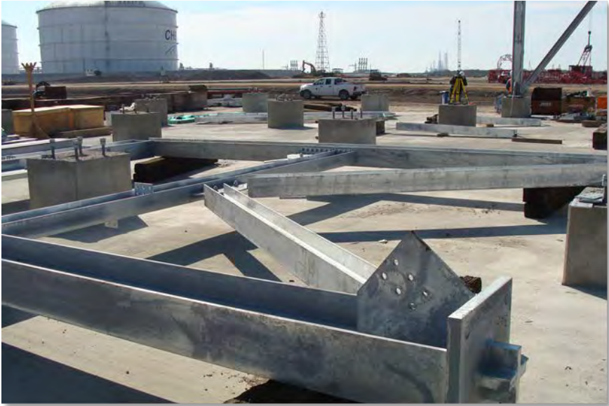
Staged Steel Area 131N (7-Mar-2013)
