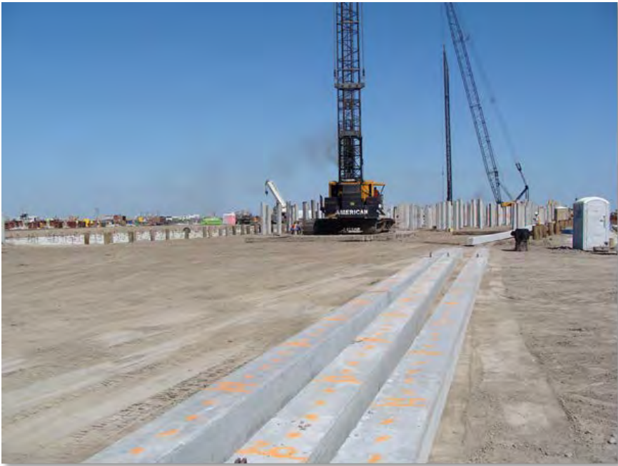
Staged and Pile Driving by BoMac (14-Mar-2013)
