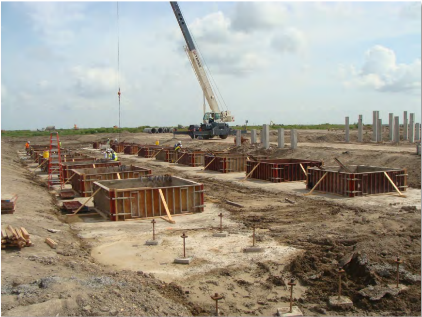
OSBL 135R03 (piperack North-South Flare) (26-July 2013)
