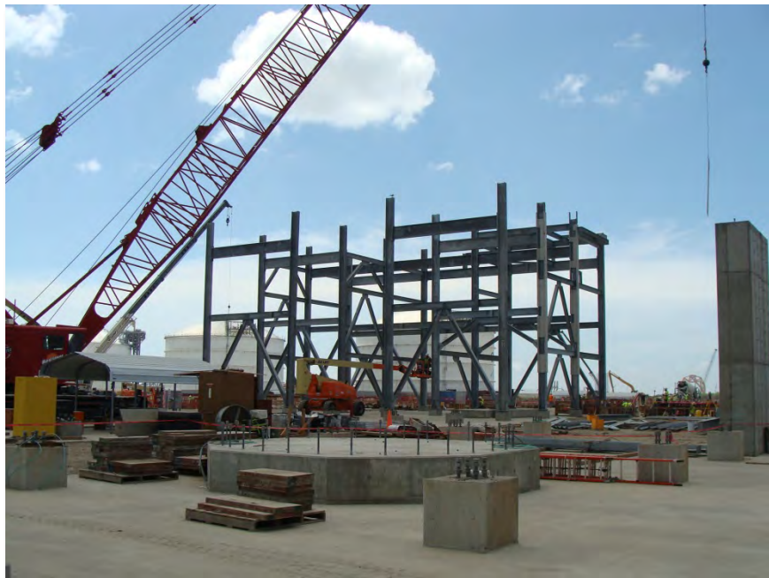
Train 1 131D (cryo air coolers piperack) (13-Aug-2013)
