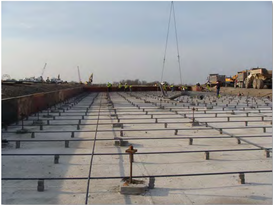
Start of Bottom Mat Rebar, Area 132N (8-Mar-2013)
