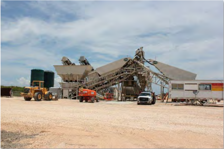
Onsite batch plant (29-July-2013)
