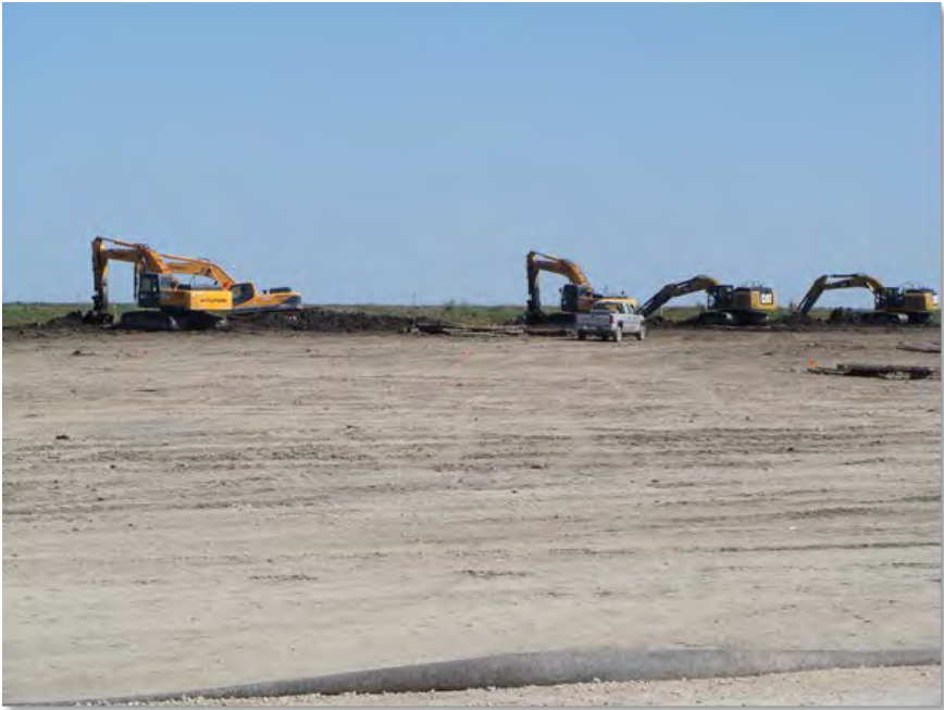
Soil Stabilization in the OSBL Area by Recon (14-Mar-2013)
