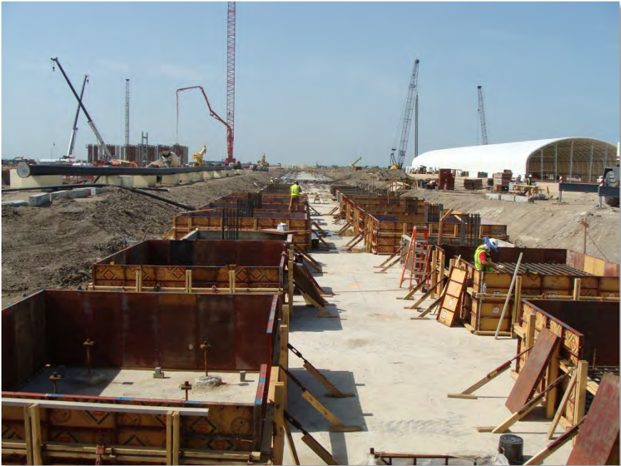
OSBL 135R01 (piperack main North-South) (29-July-2013)
