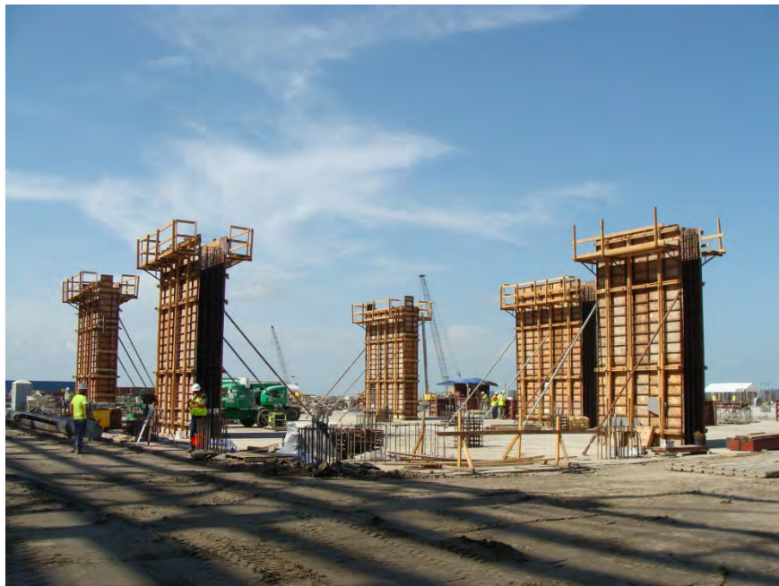
Train 1 area 131J (propane refrigeration) (18-June-2013)
