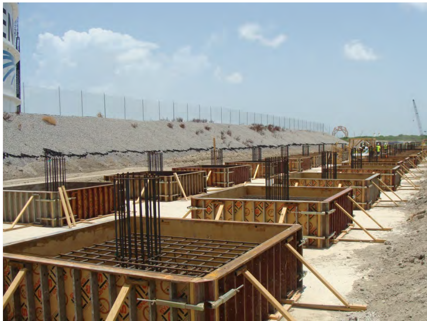
Revamp area 101R02 (Tank S-106 piperack) (20-June2013)
