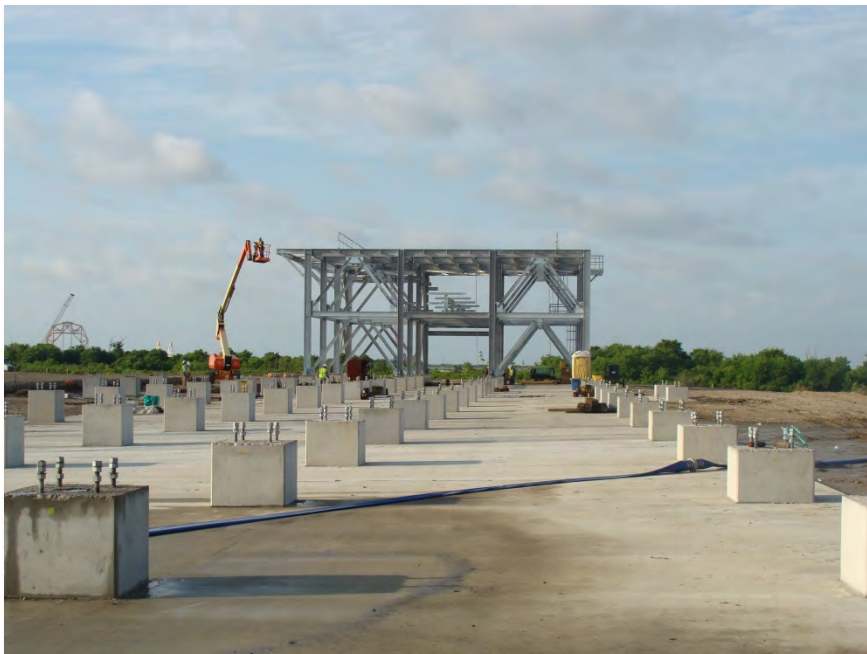
Train 2 area 132N01 (propane condenser) steel (15-May-2013)
