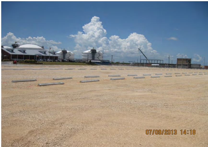
Parking Area @ Administration Building (09-July-2013)
