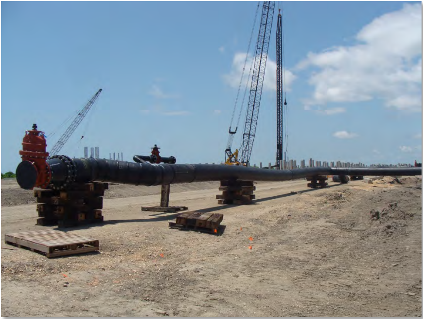
Train 1 Underground Pipe (30-Apr-2013)
