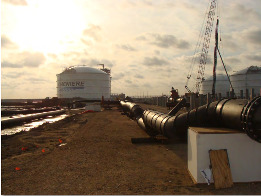
Train 1 south pipe underground HDPE (15-May-2013)
