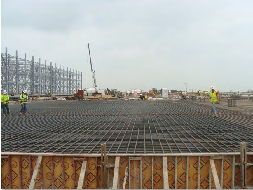
Train 1 area 131J (propane refrigeration) rebar (17-May-2013)
