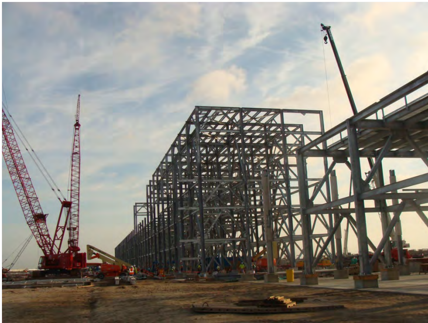
Train 1 area N01 (propane condensers) steel (15-May-2013)
