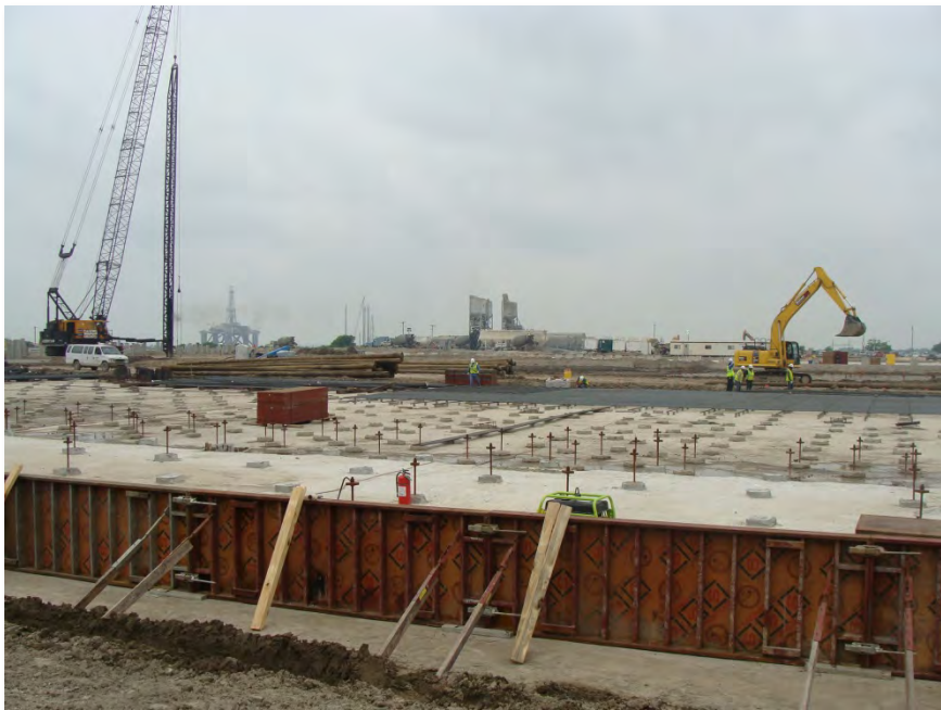
Train 2 area 132A (ethylene air compressors) center form rebar (17-May-2013)
